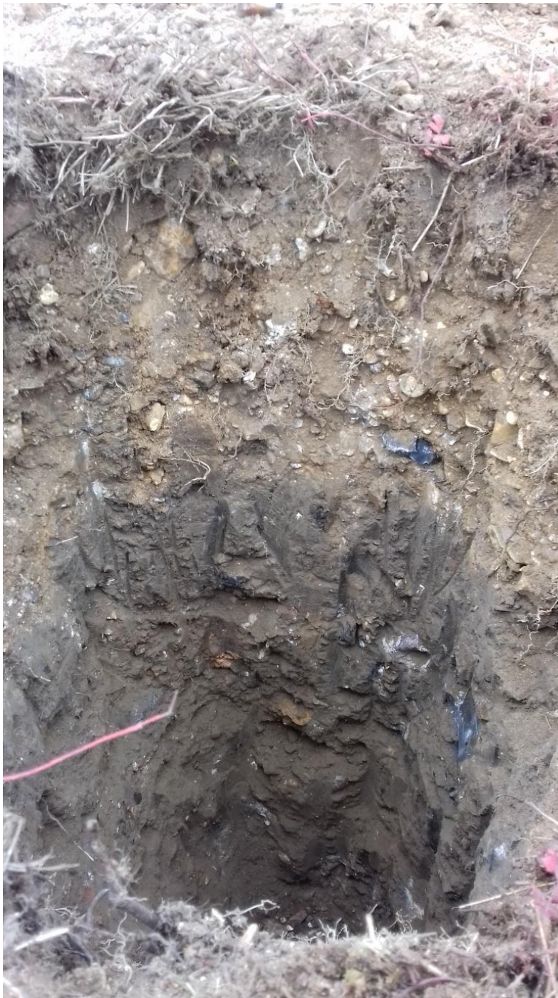
PLATE 7: HP07 SHOWING DOWNHOLE ENCOUNTERED MATERIAL.
