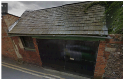
(typical older/possibly original stable/mews-like garage structure along Eldon Terrace)
