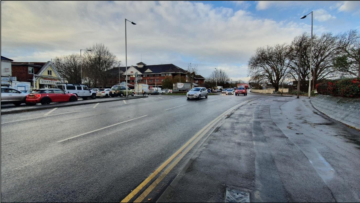
Figure 3.7 – Caversham Road north toward River Thames
