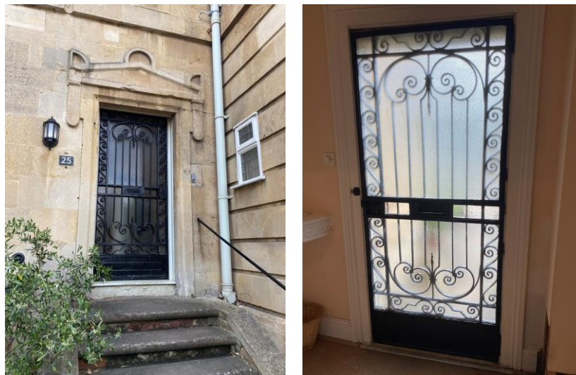
Figures 31 and 32: Existing contrasting front door viewed externally (left) and internally (right)
