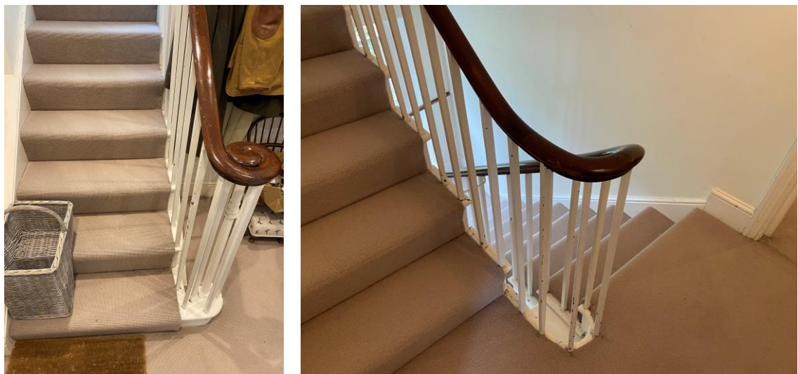
Figures 19 and 20: Altered ground floor staircase (left) and original first floor flight (right)
