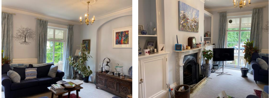
Figures 17 and 18: Main room at ground floor which retains original cornicing, joinery and fire surround
