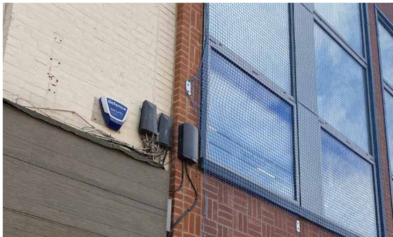
Figure 10 Photograph of existing abutment with 80 Broad Street.
