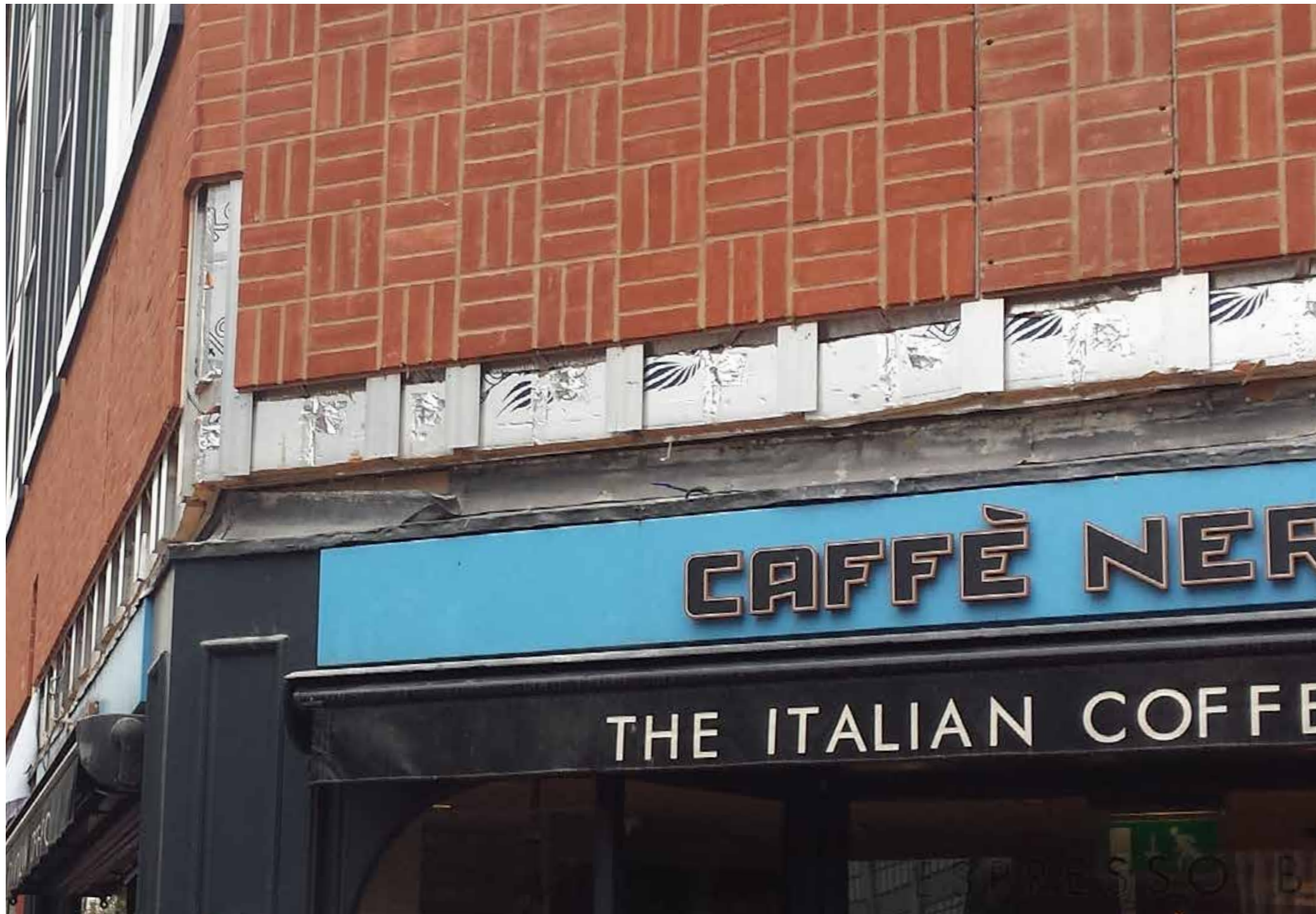
Figure 4 St Mary's House near completion showing existing cladding and phenolic Insulation
