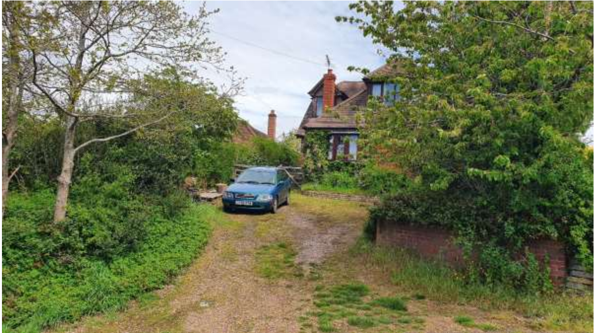
Fig. 5 – view from site entrance facing East
