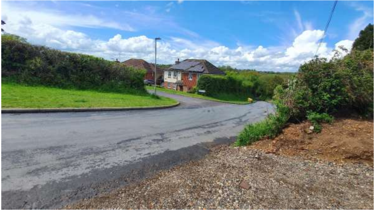
Fig. 7 – view of site entrance facing North (No. 29 tp LH side)
