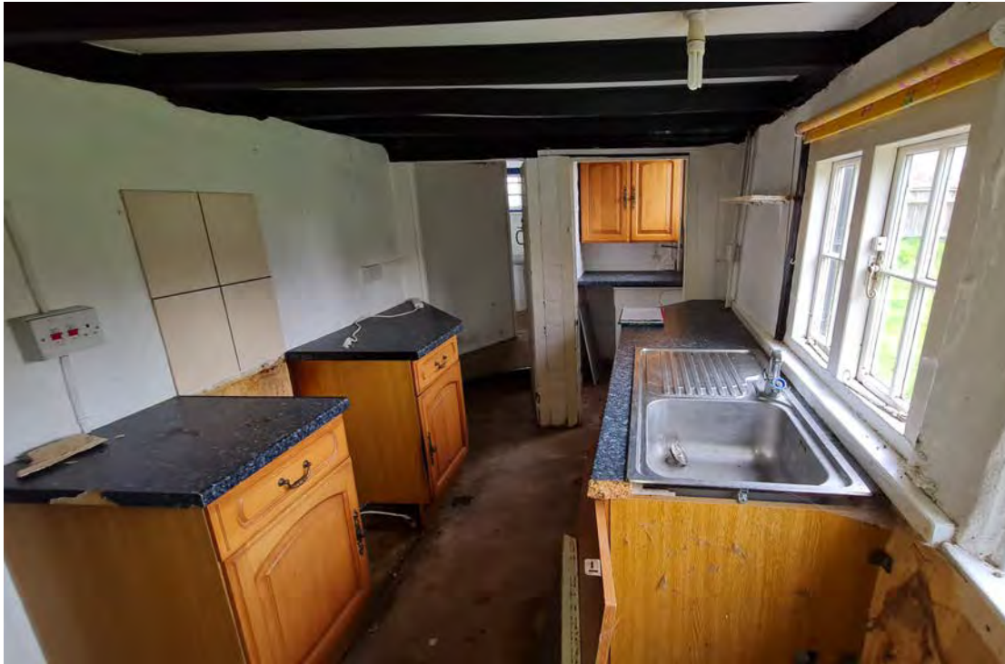
Fig 18: View of Kitchen. Note modern dividing wall on left-hand side.
