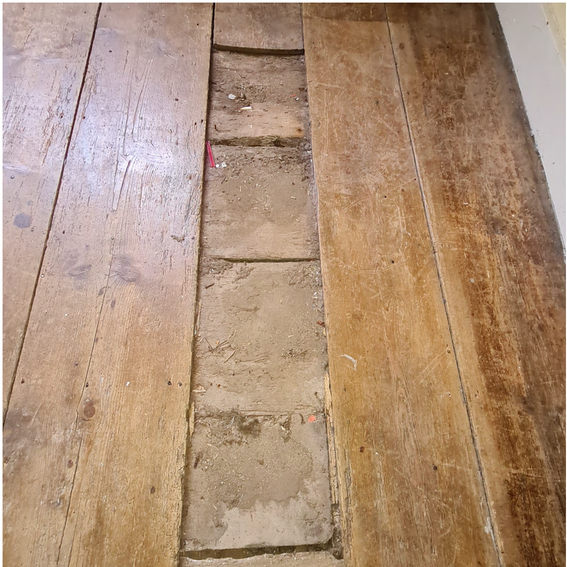
Fig 24: View of the underlying older floorboards to the first floor.
