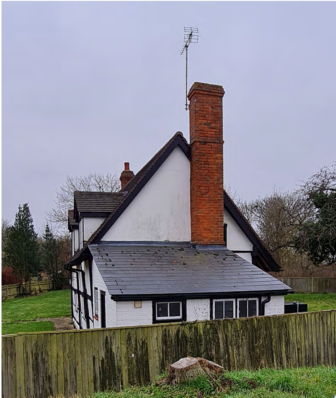
Fig 12: North-East elevation. Note again the packing-off and rendering of the gable.
