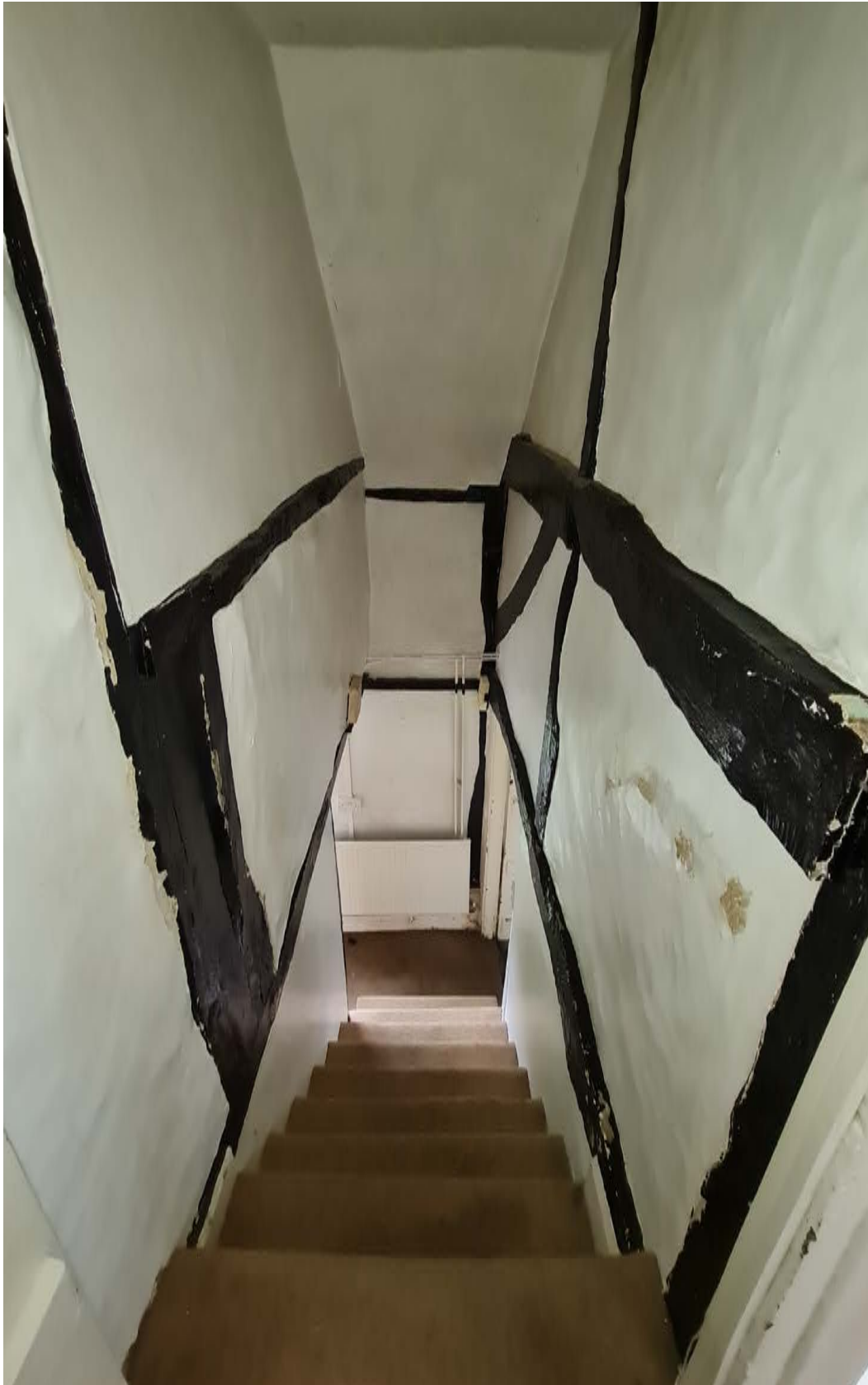
Fig 20: View of stair rising between two narrowly spaced frames.
