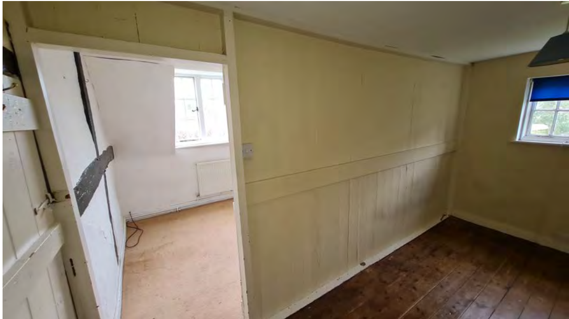
Fig 23: View of the later dividing wall between the two first floor bedrooms.
