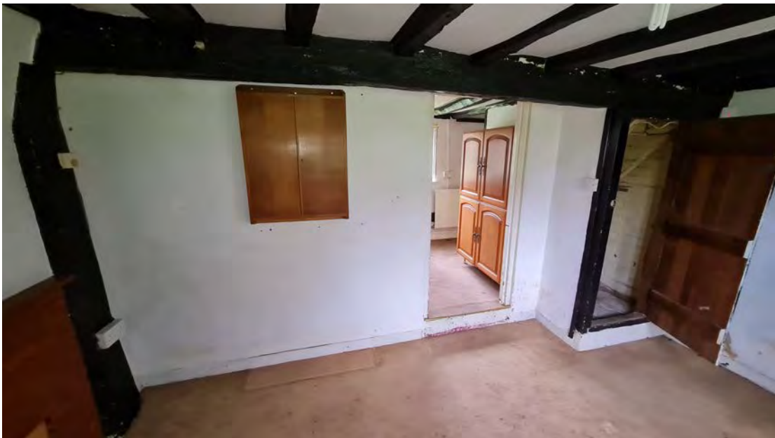
Fig 19: View of wall between Kitchen and Dining Room from Dining Room side. Note raised floor to Kitchen, which is one step higher than the rest of the ground floor.
