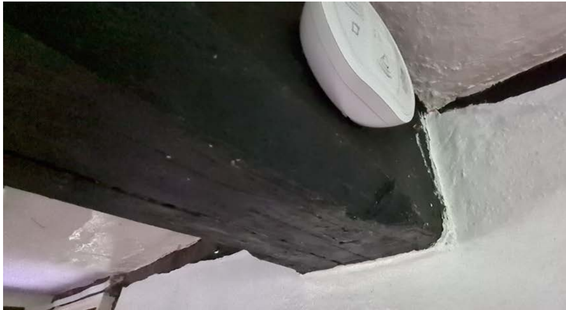
Fig 16: View of step-stop to end of axial beam in Living Room.
