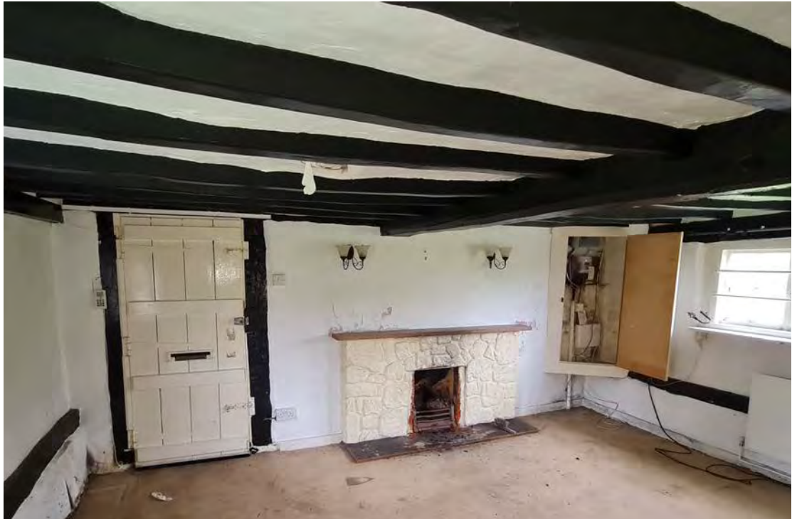
Fig 14: Internal view of the Living Room and North-Eastern fireplace. Note also the exposed floor beam and joists to the first floor.
