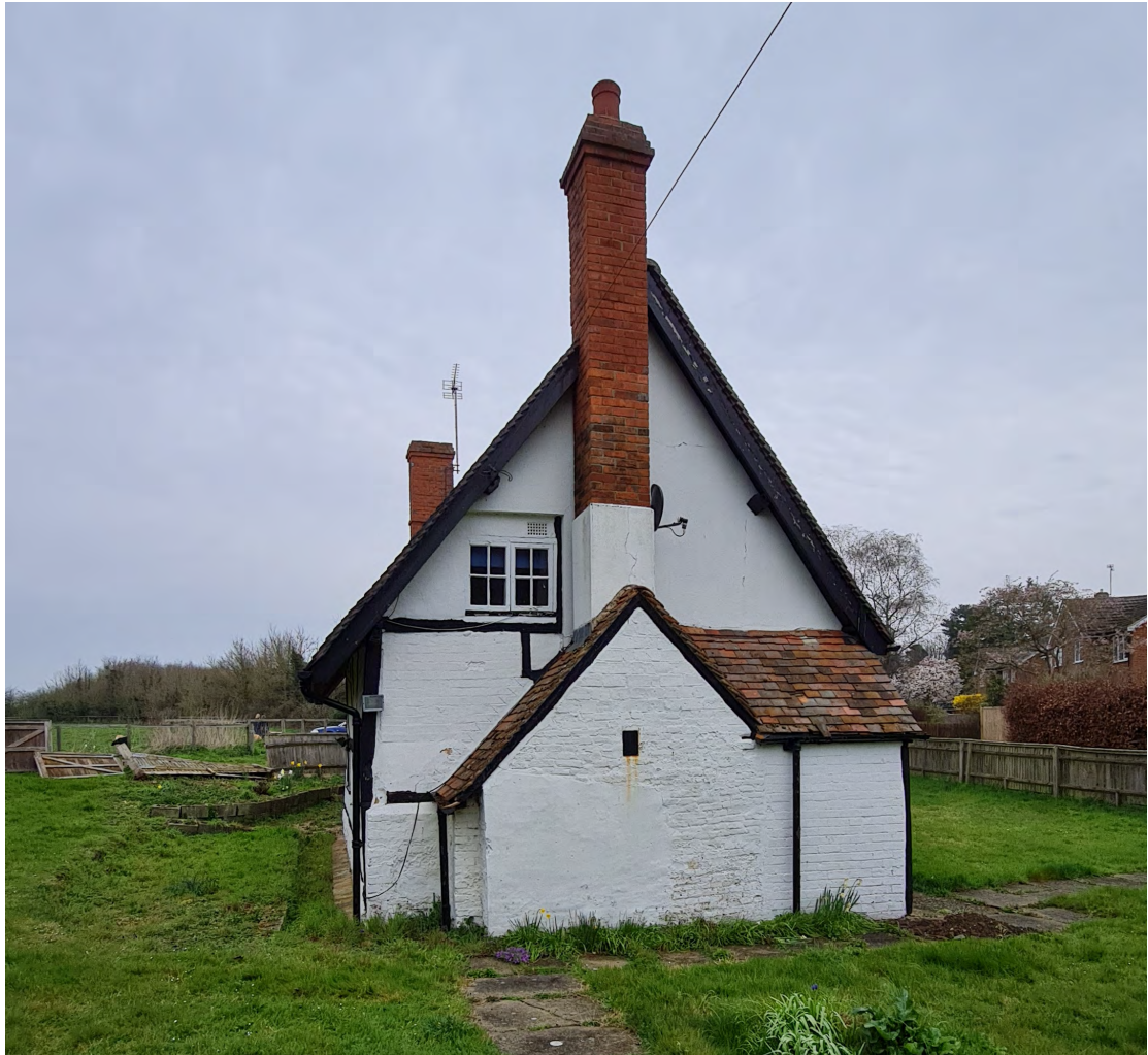
Fig 10: South-West end elevation. Note the projection for the fireplace, with chimney above built as a separate stack against, but not attached to, the gable. The projection continues as the porch to the right-hand side. Above this the wall has been packed out and rendered.
