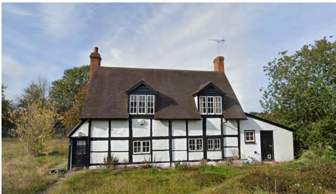
Fig 8: The South-East elevation of 3 Gravel Hill Cottages, viewed from Blagrove Lane.
