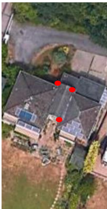
Figure 3: Location of Notable Features Identified During Dwelling External Inspection; Image Source: Google
