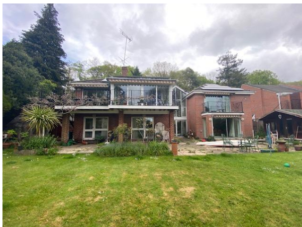
Rear elevation of dwelling
