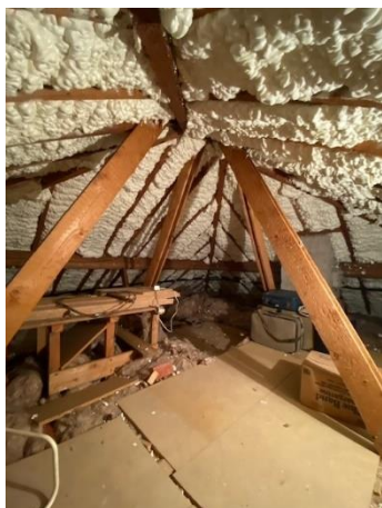
Internal western loft with foam roof space
