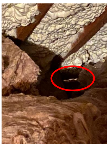
Visible light within corner of western loft space
