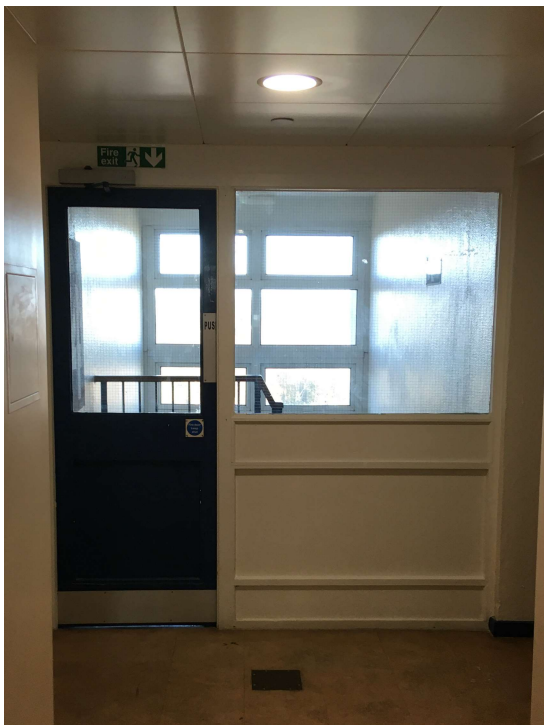
Corridor – Glazed Internal Doorset
