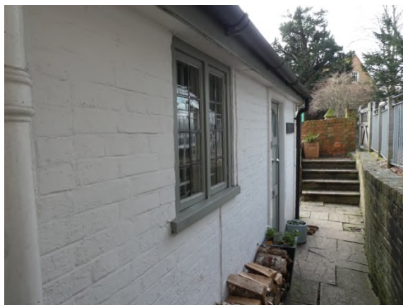
Figure 18: Right hand side of the north-west elevation with modern door to the right
