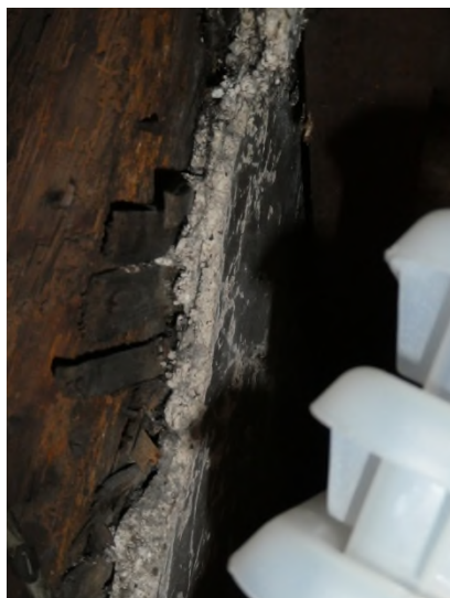
Figure 22: Lath and plaster finish on the upper part of the wall on the north-west side of the kitchen
