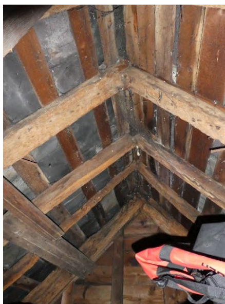
Figure 32: Mix of flatways and on-edge rafters
