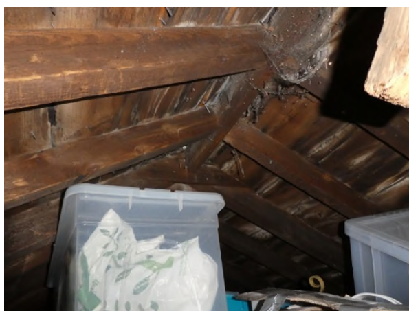
Figure 23: Roof structure over the kitchen
