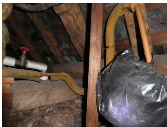
Figure 31: Clasped purlin roof structure over the first floor bedrooms
