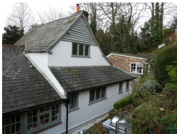
Figure 17: Phase 1 structure with 1920s lean-to
