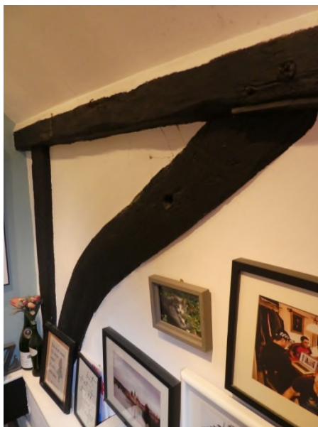
Figure 29: Ogee brace on the first floor
