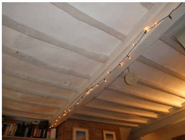
Figure 24: Chamfered beams and joists in the living room
