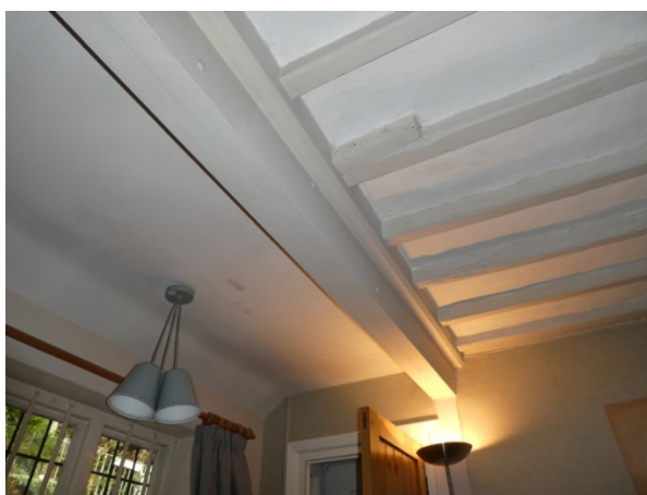
Figure 25: 1920s beam on the north-eastern side of the living room
