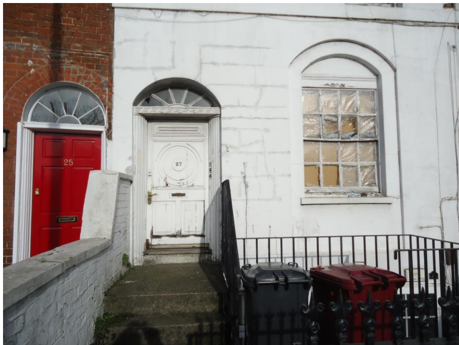
Figure 4 Image of South frontage of No 27 prior to window replacement
