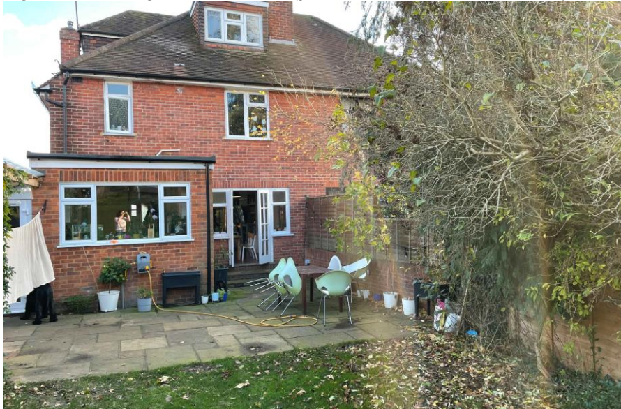
Figure 1: Existing Rear Elevation (photo received on 2 nd February 2022)
