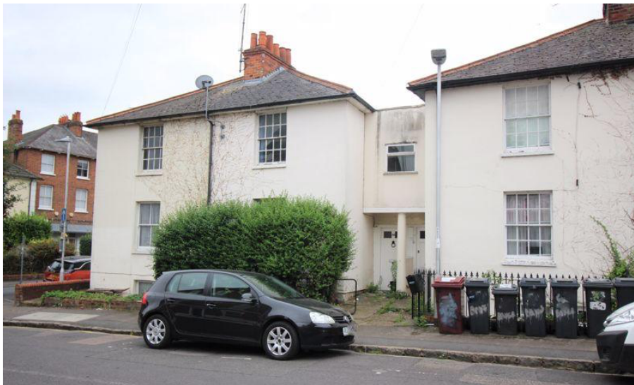
Plate 2: Front Elevation of No 33-37 Baker Street (No 35 has the hedge, window above entrance is to be replaced)
