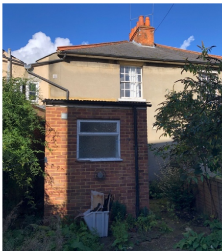
Plate 3: Rear elevation of No.35 with brick built single-storey extension
