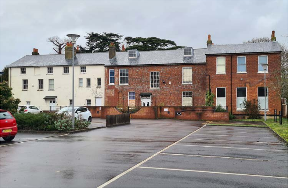
Plate 3.2 Rear elevation, Yeomanry House
