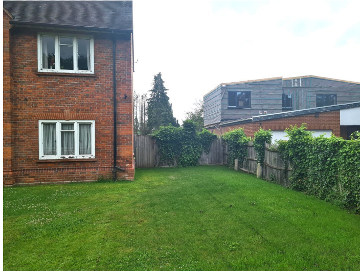
131 Whiteknights Road, first floor extension under construction, June 2021
