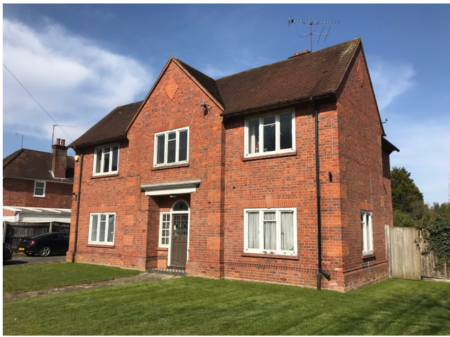
Front elevation showing fine brick detailing and simple geometry
