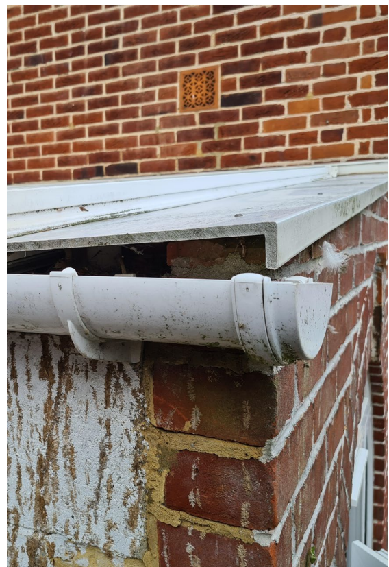
127 Whiteknights Road lean-to roof over garage and store. As this space is unheated, evidenced by the uninsulated roof, it could not be considered a habitable room, as confirmed by the owner.
