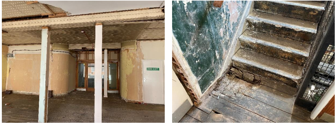
Figures 33 and 24: Curved partitions at first floor and a view of the 1930s stair and lift core located to the rear of the building
