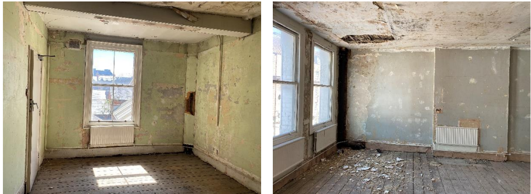
Figures 35 and 36: Internal views within 147 Friar Street showing surviving partitions and chimney breasts
