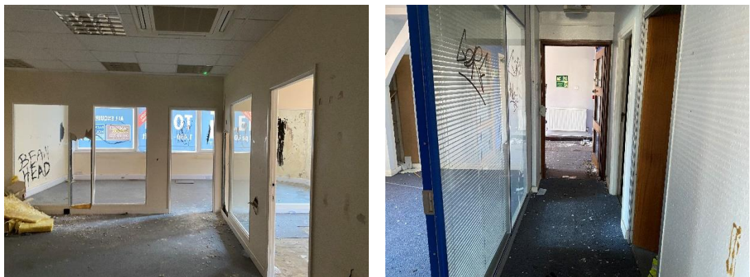
Figures 24 and 25: Open plan layout and modern partitions present within 1-3 Queen Victoria Street and 148 Friar Street
