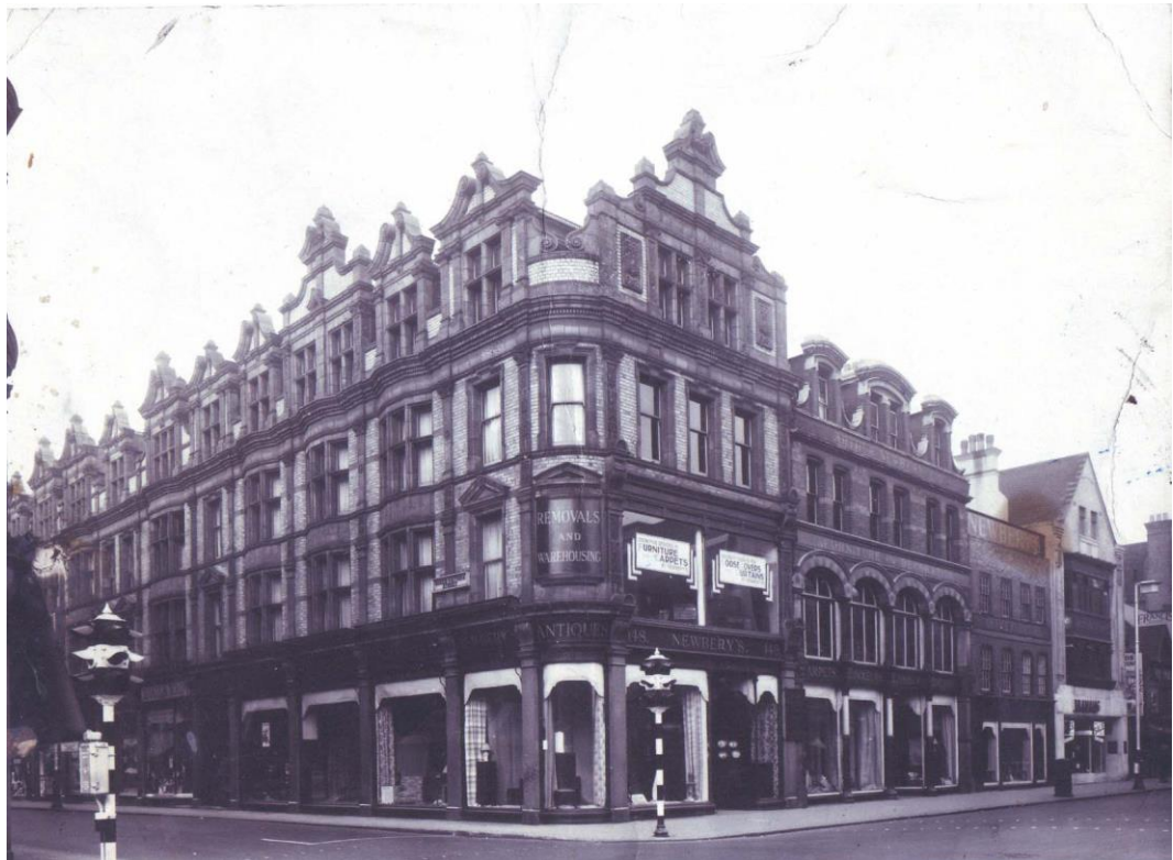
Figure 11: 1939 Photograph of the site when it was in use as Newbery's Furniture Store
