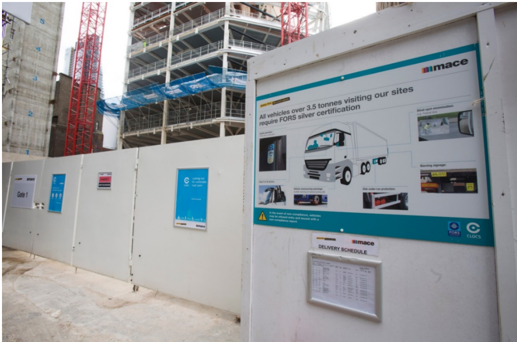
Figure 5.1: Example Site Hoarding
