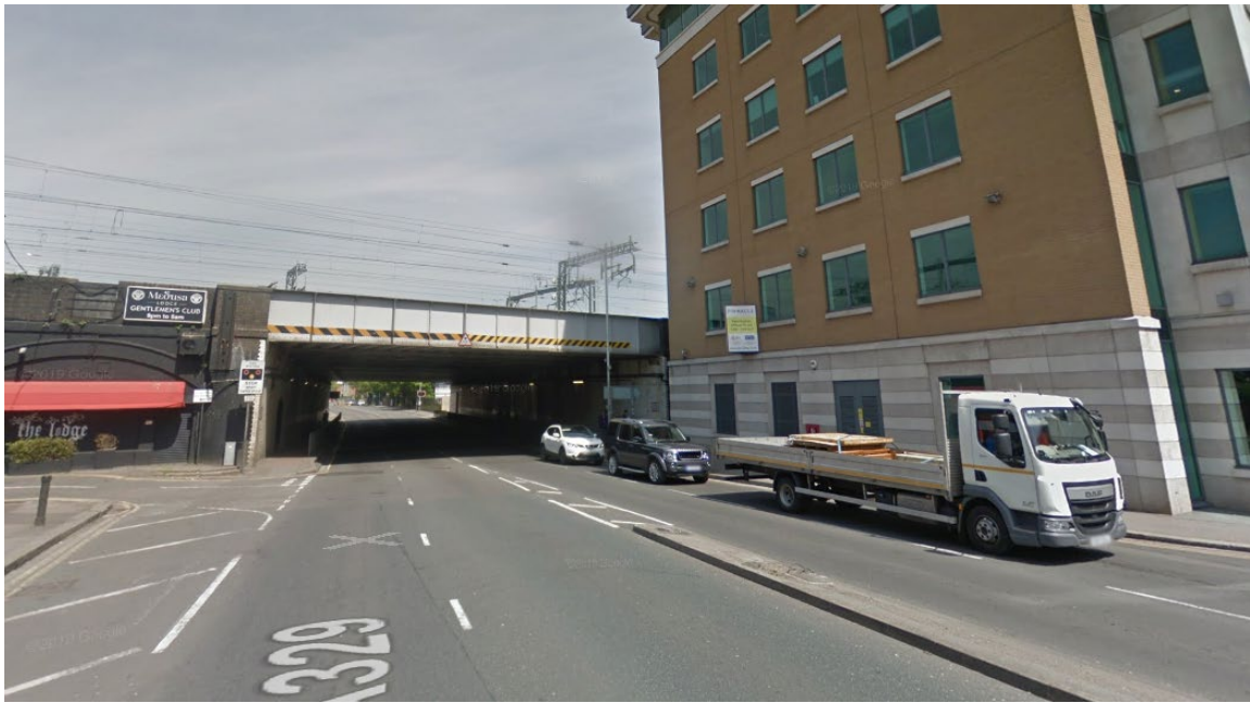
Figure 5.3: Railway Bridge on A329
