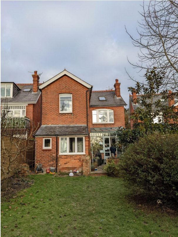
Rear elevation showing lean to extension and conservatory
