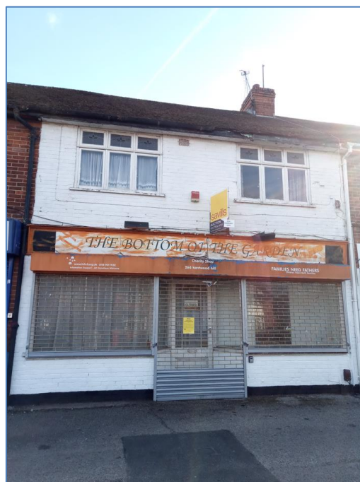
Fig 2 - Photograph of the existing front of 264 Kentwood Hill taken by case officer on 09/02/2022
