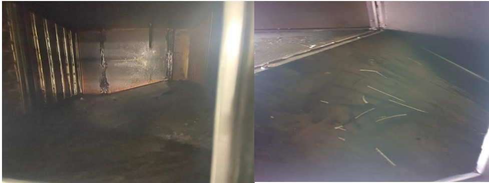
Typical Ductwork after cleaning
