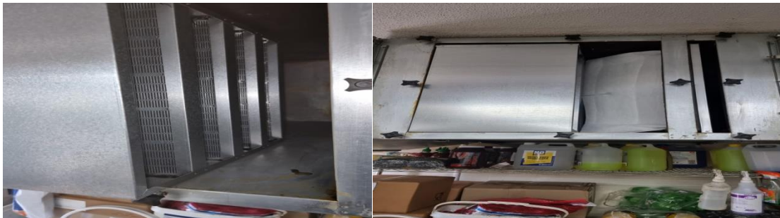
Filter housing and filters after cleaning - changing
