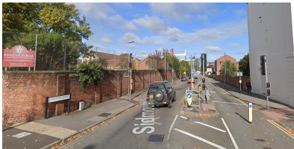
Dedicated cycle lanes along Sidmouth Street
