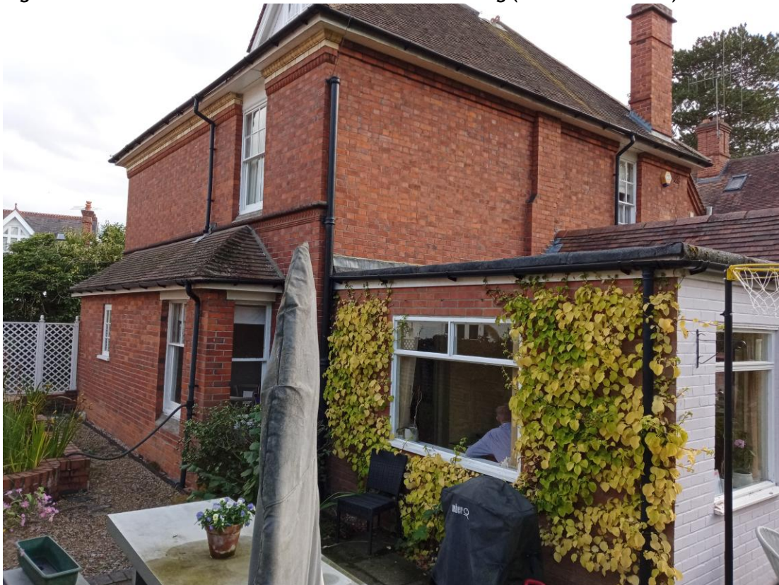
Figure 3: Existing North-east elevation (Site Visit 4/10/22)
