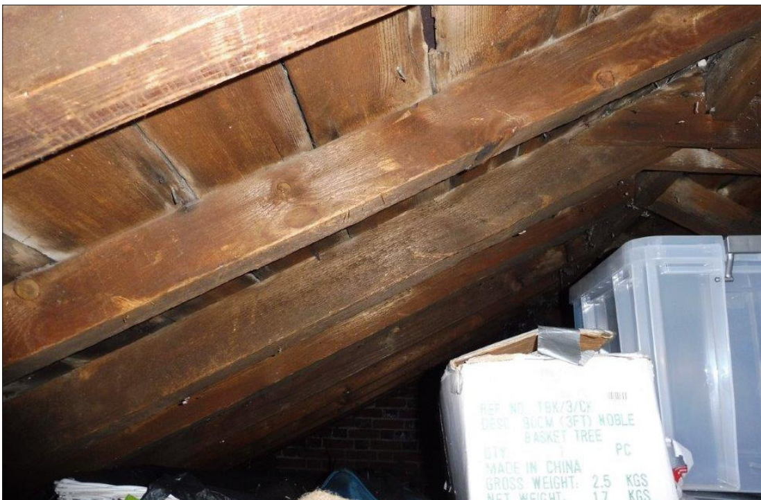
PHOTOGRAPH 2: Loft Void within Building B1a
