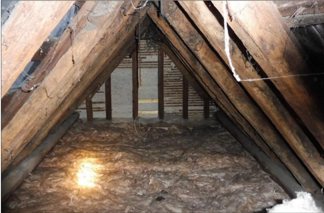
PHOTOGRAPH 3: Loft Void within Building B1b
