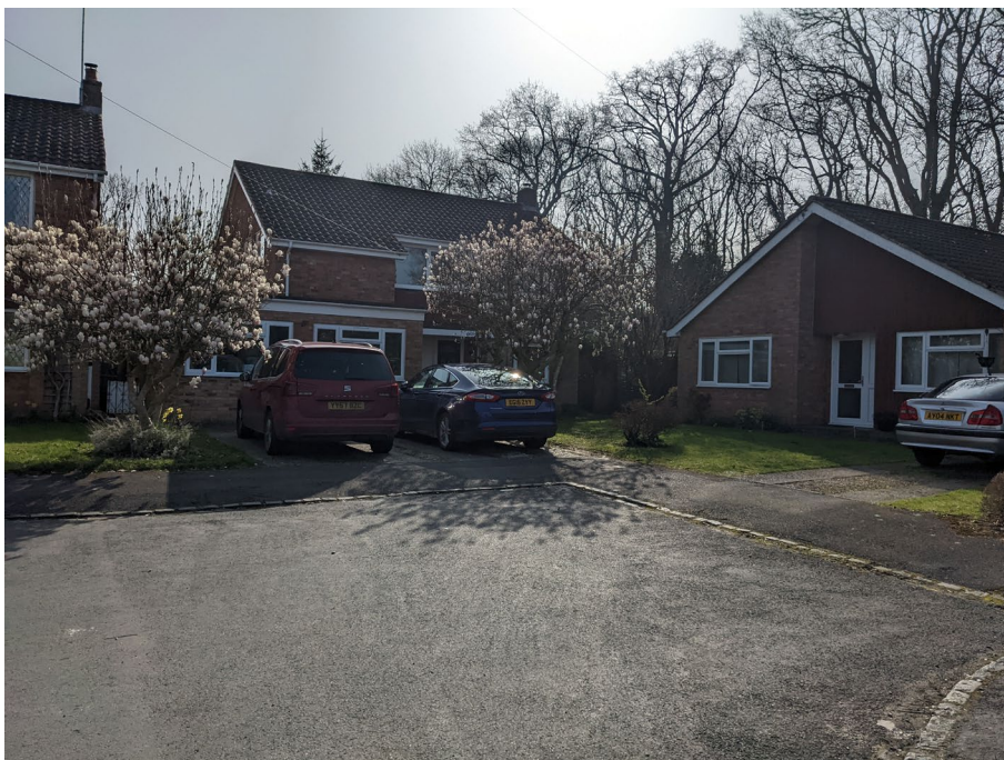
Front elevation showing 16 Tower Close (left hand side) and 17 Tower Close
