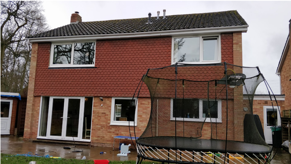
Rear elevation showing 16 Tower Close
