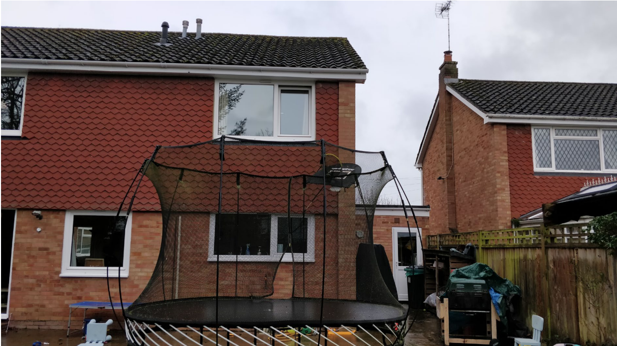
Rear elevation showing 16 Tower Close and 15 Tower Close adjacent
