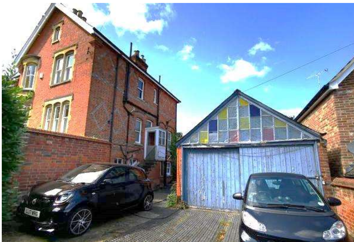
Plate 2: External view looking southwest to towards the east elevation of the garage in relation to the northeast elevations of the house
