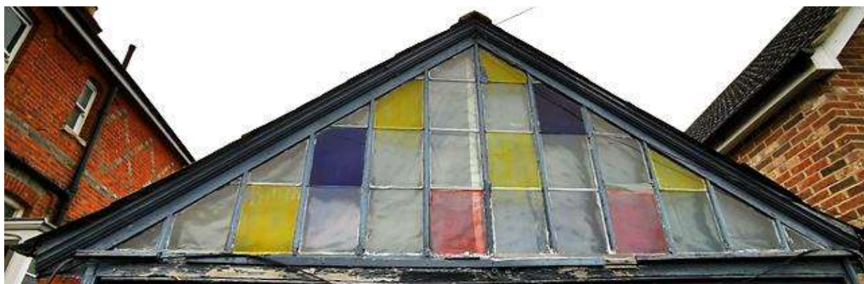
Figure 3: External view looking west towards the upper east elevation showing timber framed glass in detail
