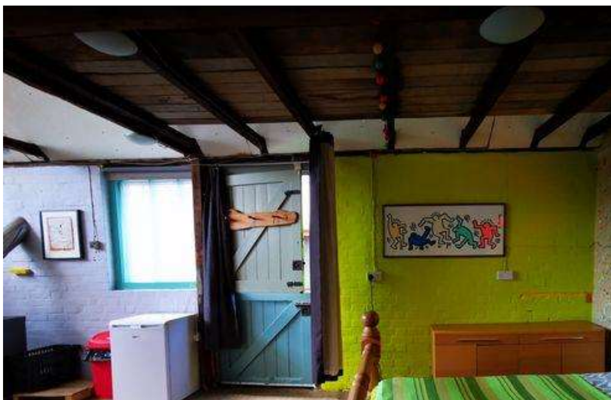
Plate 10: Internal view of the south elevation
