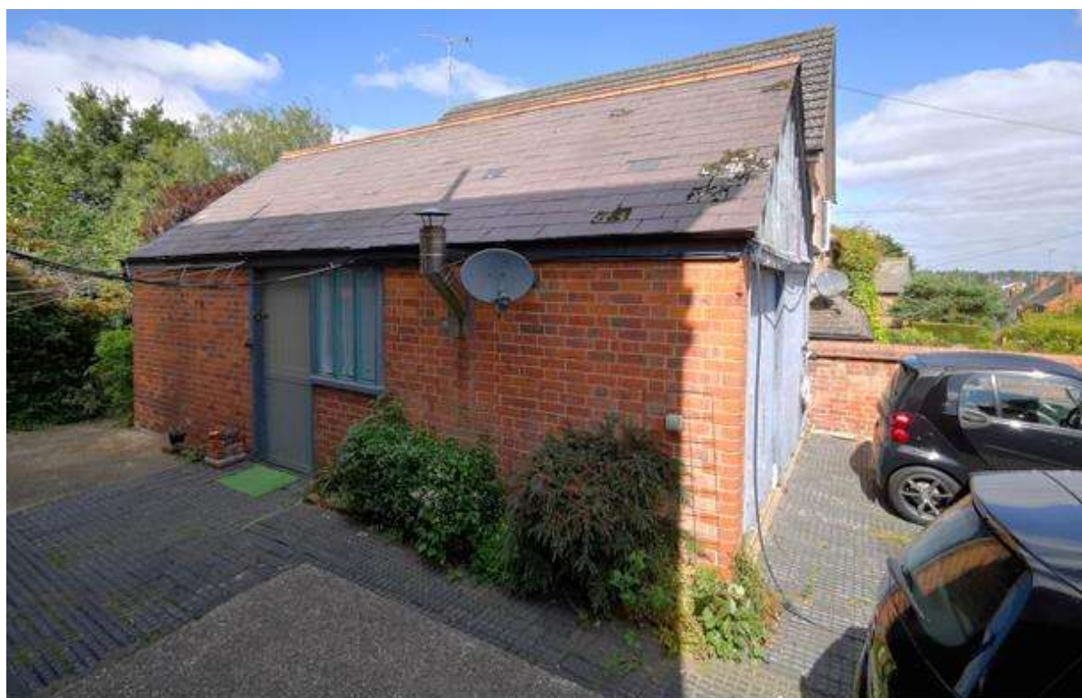
Plate 6: External view looking northwest towards the south elevation and the roof of the garage
