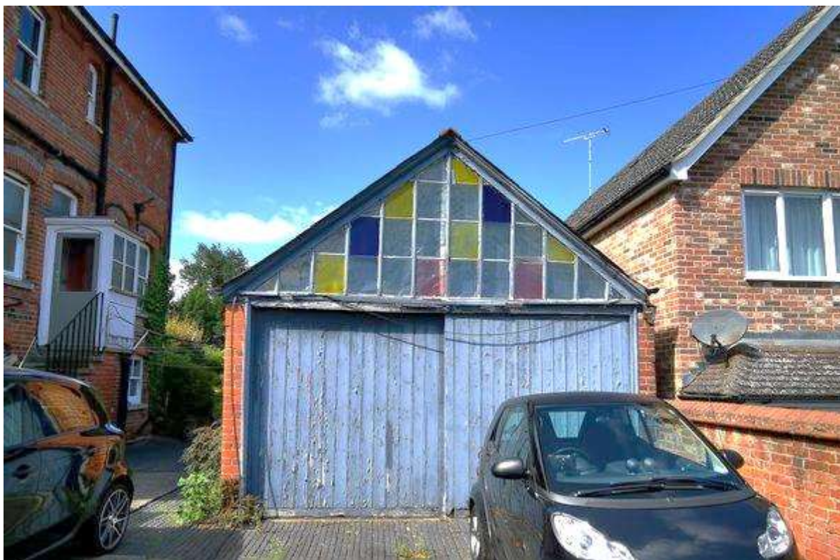
Plate 1: External view looking west to the east elevation
