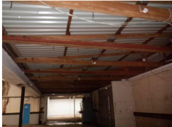
18. Northern side open to the roof with underside of corrugated metal sheeting visible (B1)
