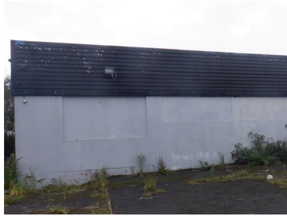
8. Flat roof on the rear elevation of the showroom (B1)
