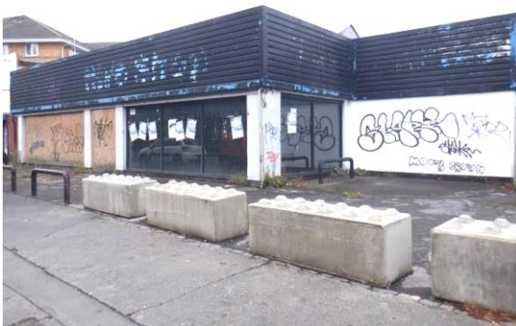
5. Showroom building, viewed from the south (B1)
