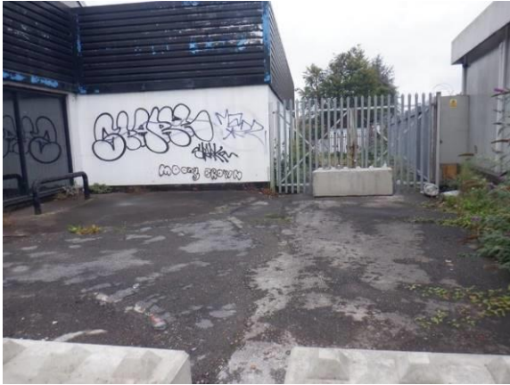
1. Asphalt hard standing to the southern side of the site (OH1)
