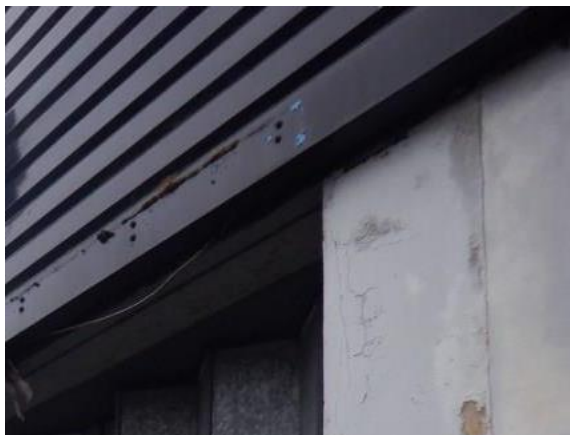
10. Metal panelling tight to blockwork, eastern elevation (B1)
