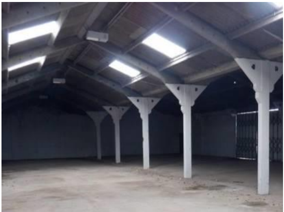
29. Corrugated asbestos roofing visible, with clear corrugated plastic skylights (B3)
