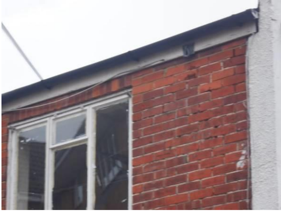
19. Flat roof office tight to the fascia, viewed from the south-west (B2)
