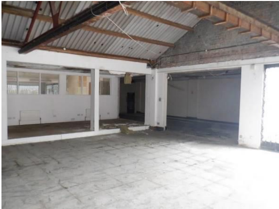
13. Internal of the showroom, open to the ceiling with metal rafters and underside of roofing visible (B1)
