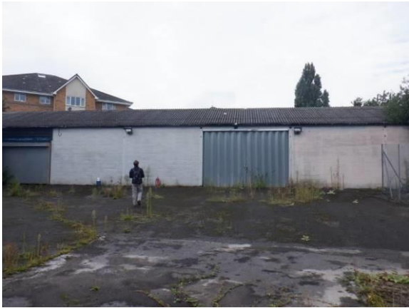
7. Warehouse, viewed from the east (B3)
