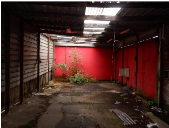
21. Covered storage yard (B2)
