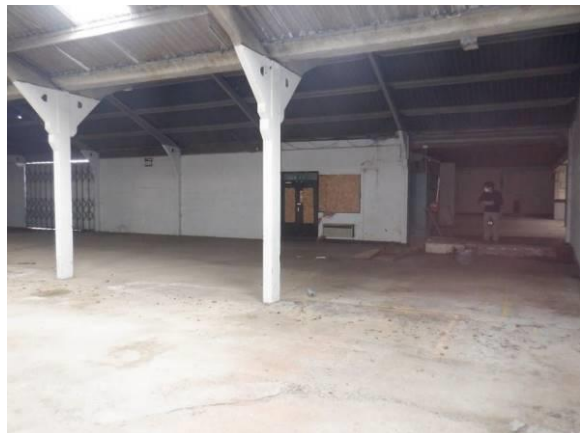
28. Concrete floor throughout the internal of the warehouse (B3)
