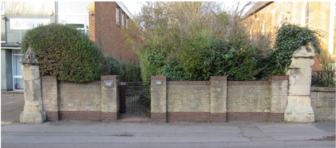
Fig.50: Photograph of existing Oxford Road boundary treatment
