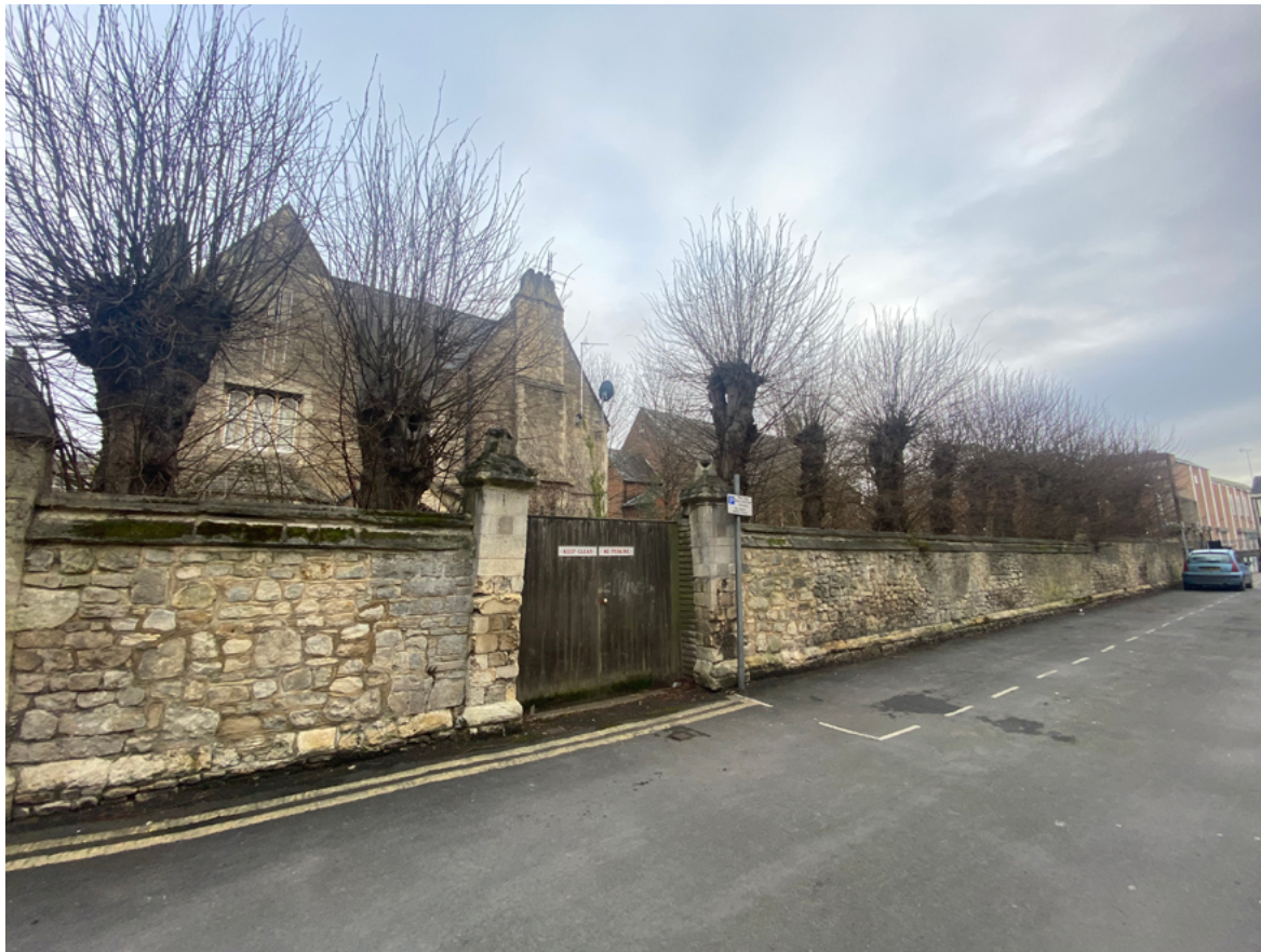
Fig.52: Photograph of existing vehicle access gates
