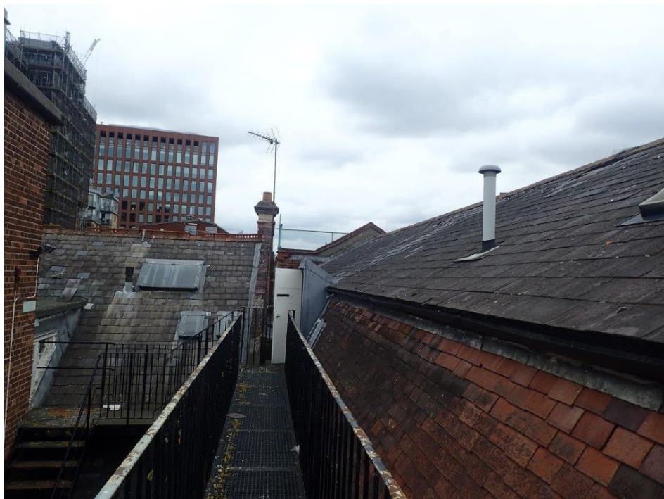
Photograph 4: Roof of buildings on the site.
