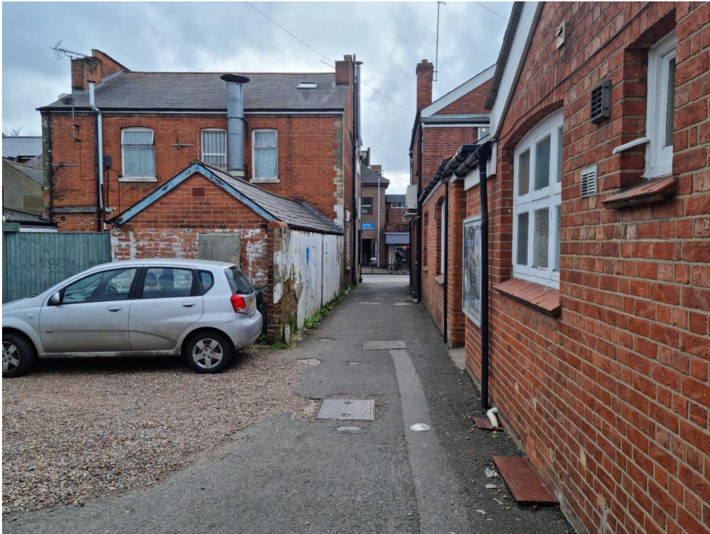
Photo 5: Side Lane and rear of application site, facing south
