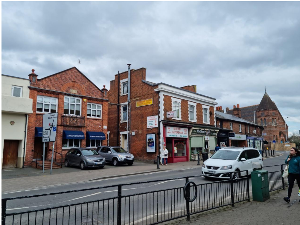
Photo 2: Application site frontage, facing NE
