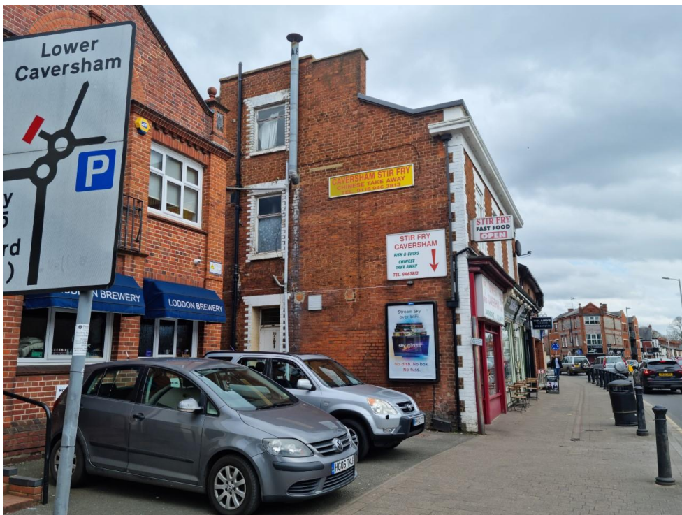
Photo 3: Weste elevation of application site, facing east
