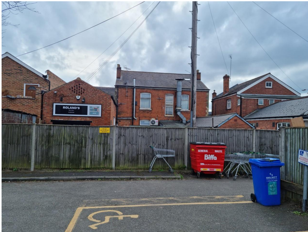
Photo 6: Rear of application site, taken from the Car Park, facing south
