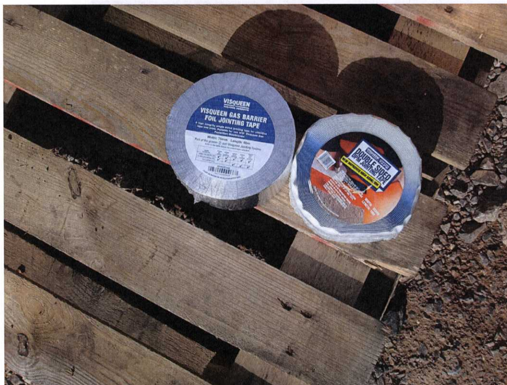
Materials used in Landgas Mitigation Measures- 20 th May 2009
