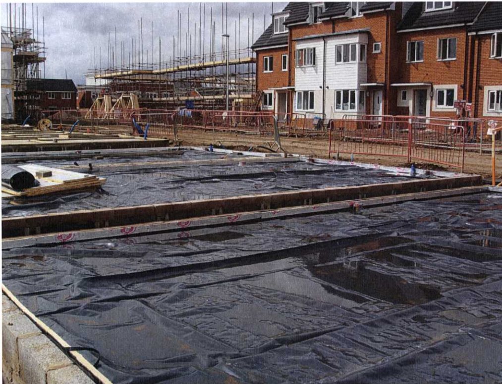
Block N Landgas membrane- 7 th September 2010
