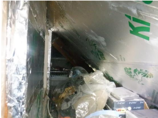
15. Eave space insulated with hard foam.
