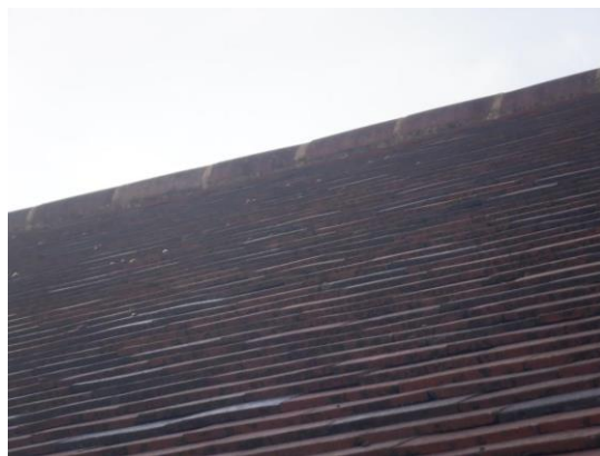
8. Fully mortared ridge tiles (front elevation).
