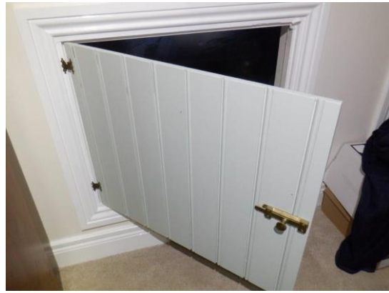
14. Cupboard eave spaces.
