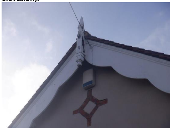
9. Ornate timber fascia and intact gable end verge mortar (front elevation).
