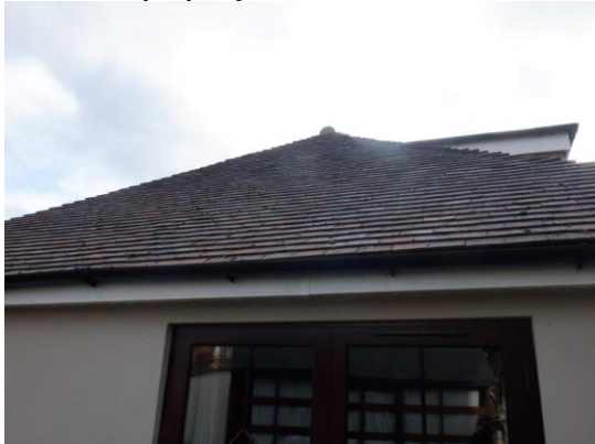
3. Mostly flat overlapping roof tiles (northern elevation).
