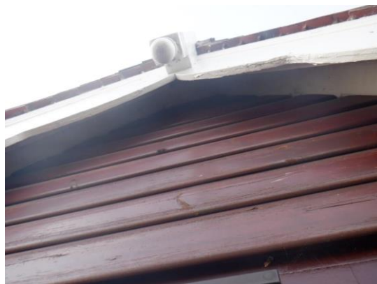
10. Tight cladding on smaller gable end (front elevation).
