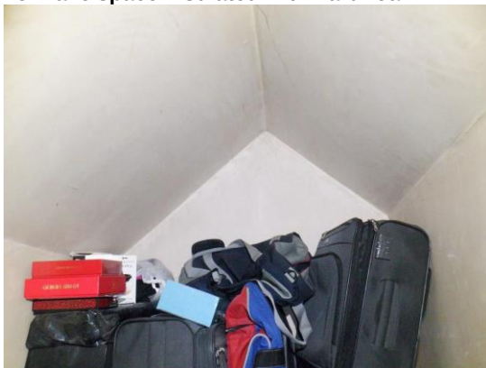
17. Front gable end storage cupboard.
