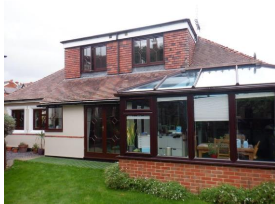
2. Rear of property viewed from west.
