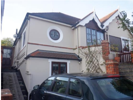
1. Front of property viewed from southeast.
