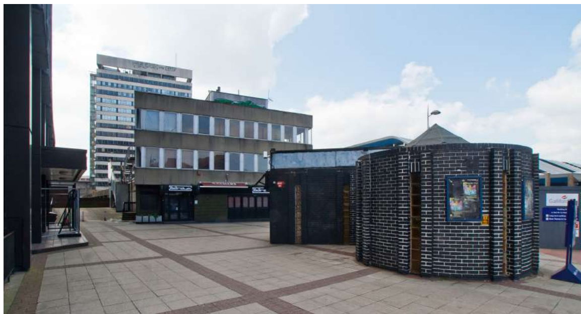
Existing Station Hill
