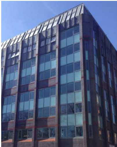
Refurbishment at One Valpy Street
