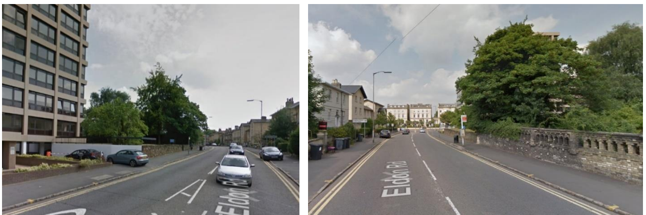
Figure 4: Views of the site from Eldon Road, when approached from the north and south.
