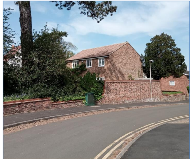
Fig 2. Rear and side of 20 Lancaster Close. Photo taken by case officer on 20/04/2022.
