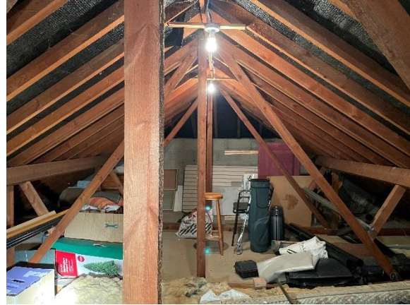
Photograph 14. The eastern loft space within the garage.
