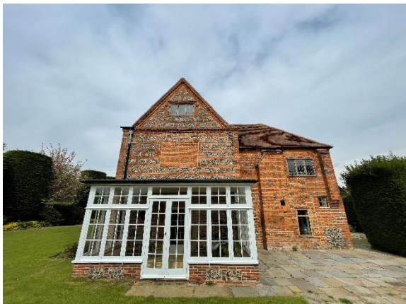
Photograph 3. The southern elevation of Old Grove House.
