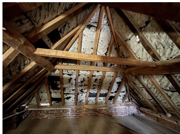
Photograph 6. The central loft space of Old Grove House.
