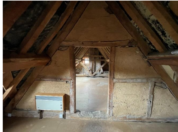
Photograph 8. The central loft space of Old Grove House.
