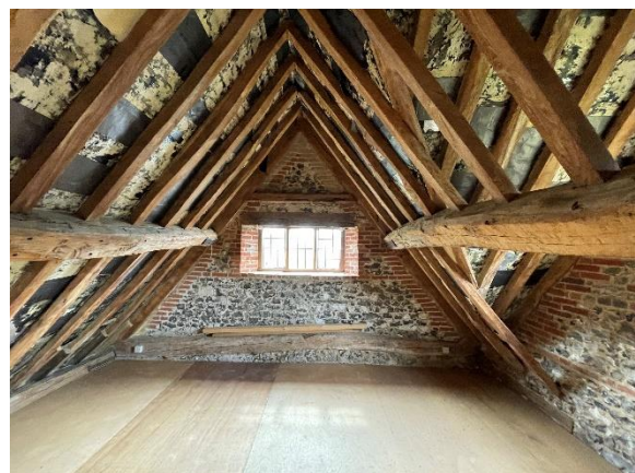
Photograph 10. The central loft space of Old Grove House.
