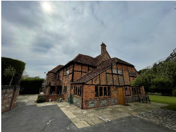
Photograph 1. The northern elevation of Old Grove House.
