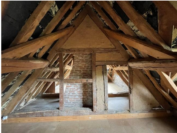
Photograph 7. The central loft space of Old Grove House.
