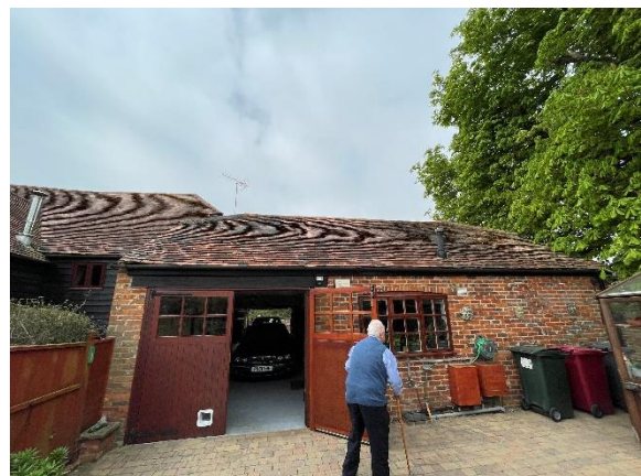
Photograph 12. The eastern elevation of the garage.
