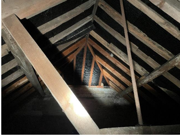
Photograph 13. The western loft space within the garage.
