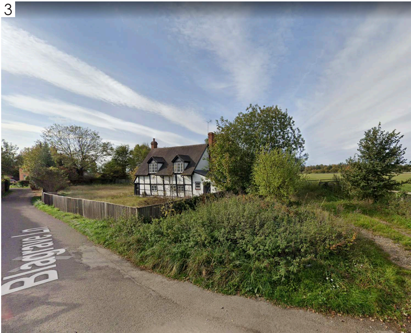
Existing view of 3 Gravel Hill Cottages with fields beyond to West. Source: Google Street View.
