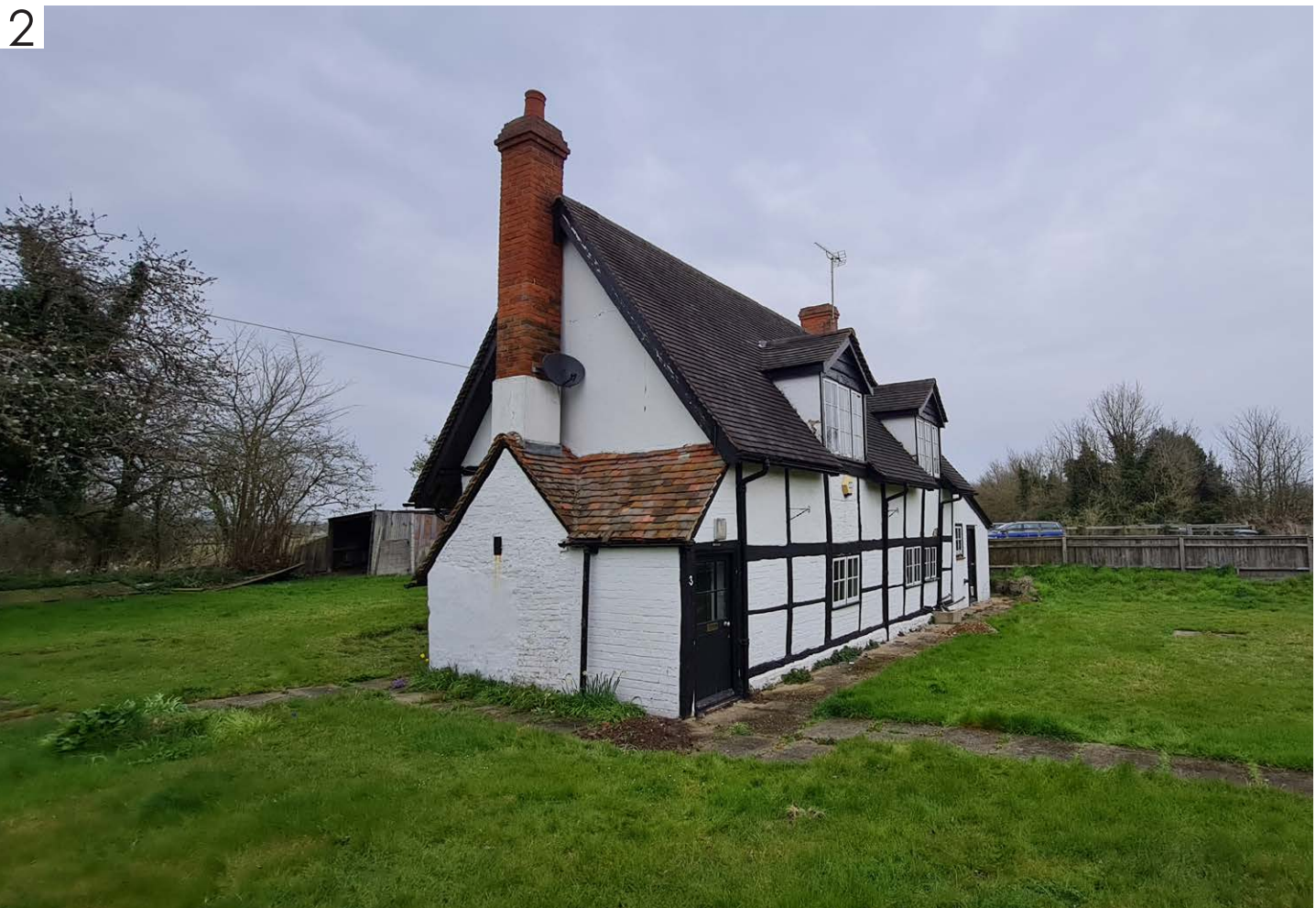
View of front and end elevations of 3 Gravel Hill Cottages, looking North.
