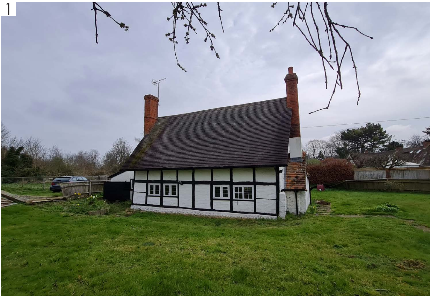
View of rear (North-West) elevation of 3 Gravel Hill Cottages.
