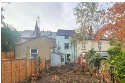
Rear of 17 St James Street
