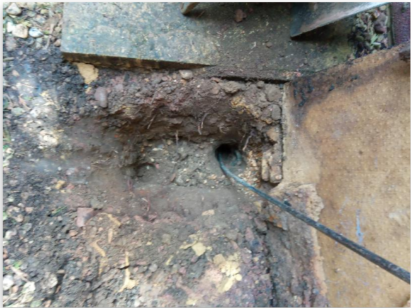
Fig 2.2: Trial Hole 2 Footing
