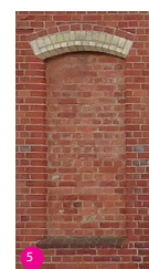
Recessed brick to mock window openings
