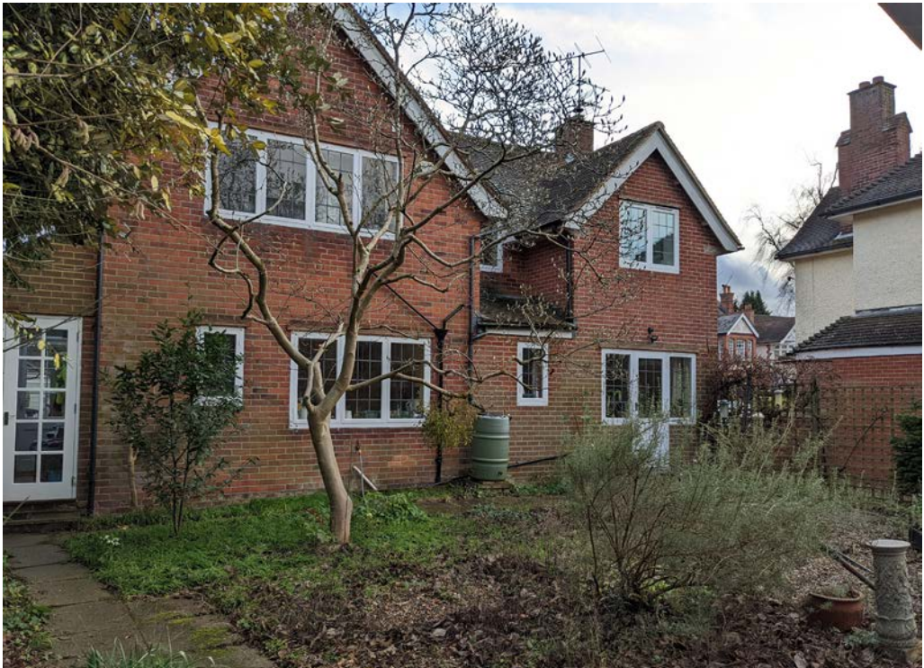
View to towards rear elevation from north east
