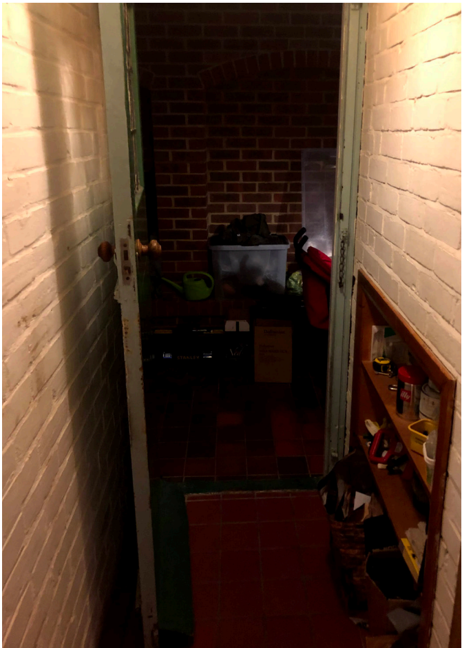
View to boot room from Kitchen
