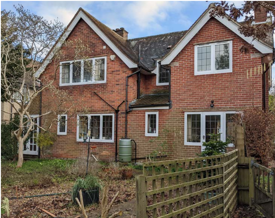
View to towards rear elevation from garage
