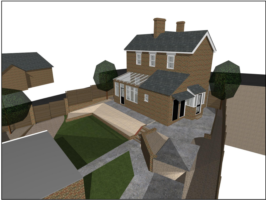
1 Existing Rear View
