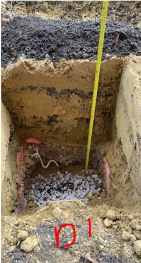
Trial pit in location D1. The contractor has reinstated the geotextile membrane on backfilling.
