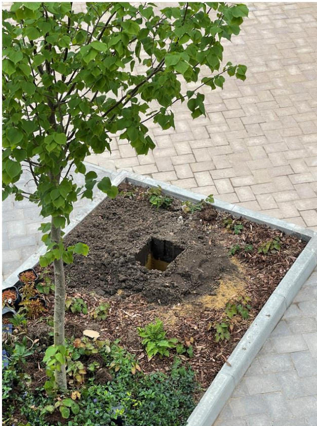
Trial pit location in square B2, demonstrating compliance with the specification.
