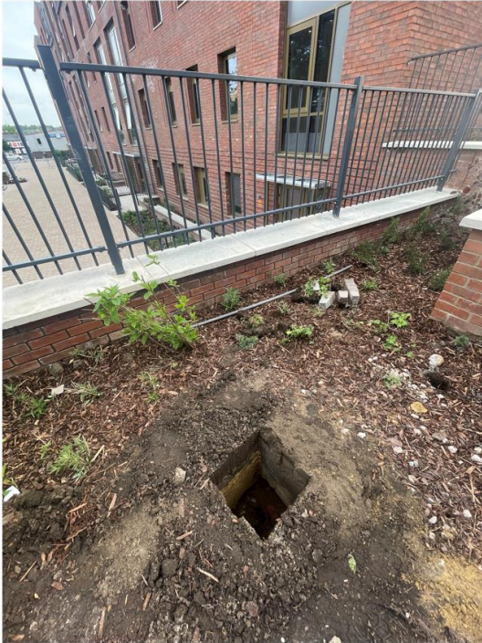
Additional Trial pit excavation at locations B1 and C1 where trial pits met the specification
