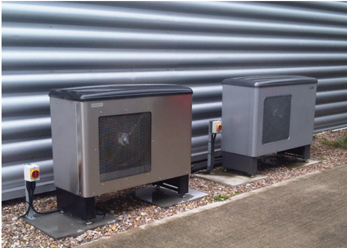
Figure 3 - Air Source Heat Pumps
