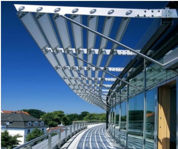
Figure 5 - Solar PV Louvres on the South Facade
