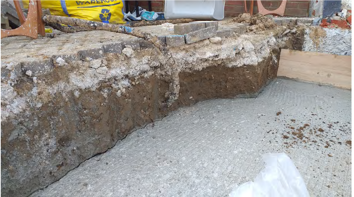
Above, the southern excavation face of the over excavated foundation in the borehole BH8 area (note wrapped cable)
