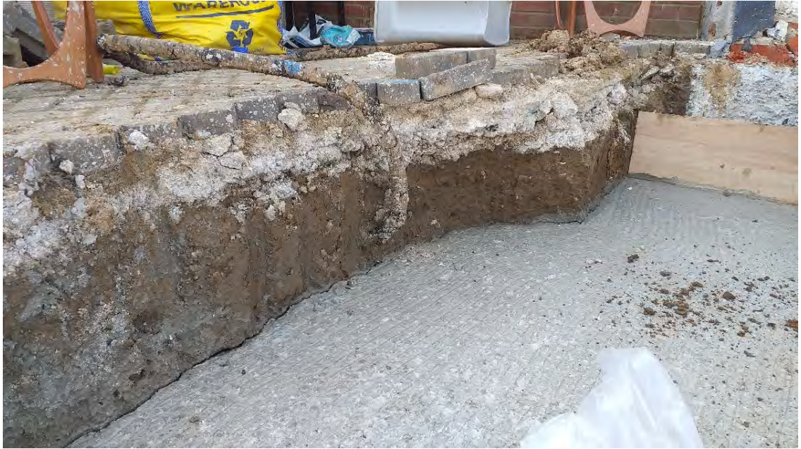
Above, a view looking south west at the edge or the widened foundation excavation in the BH8 area (note old bitumen wrapped electrical cable)
