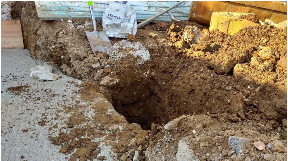
Above, excavation of the borehole BH8 location
