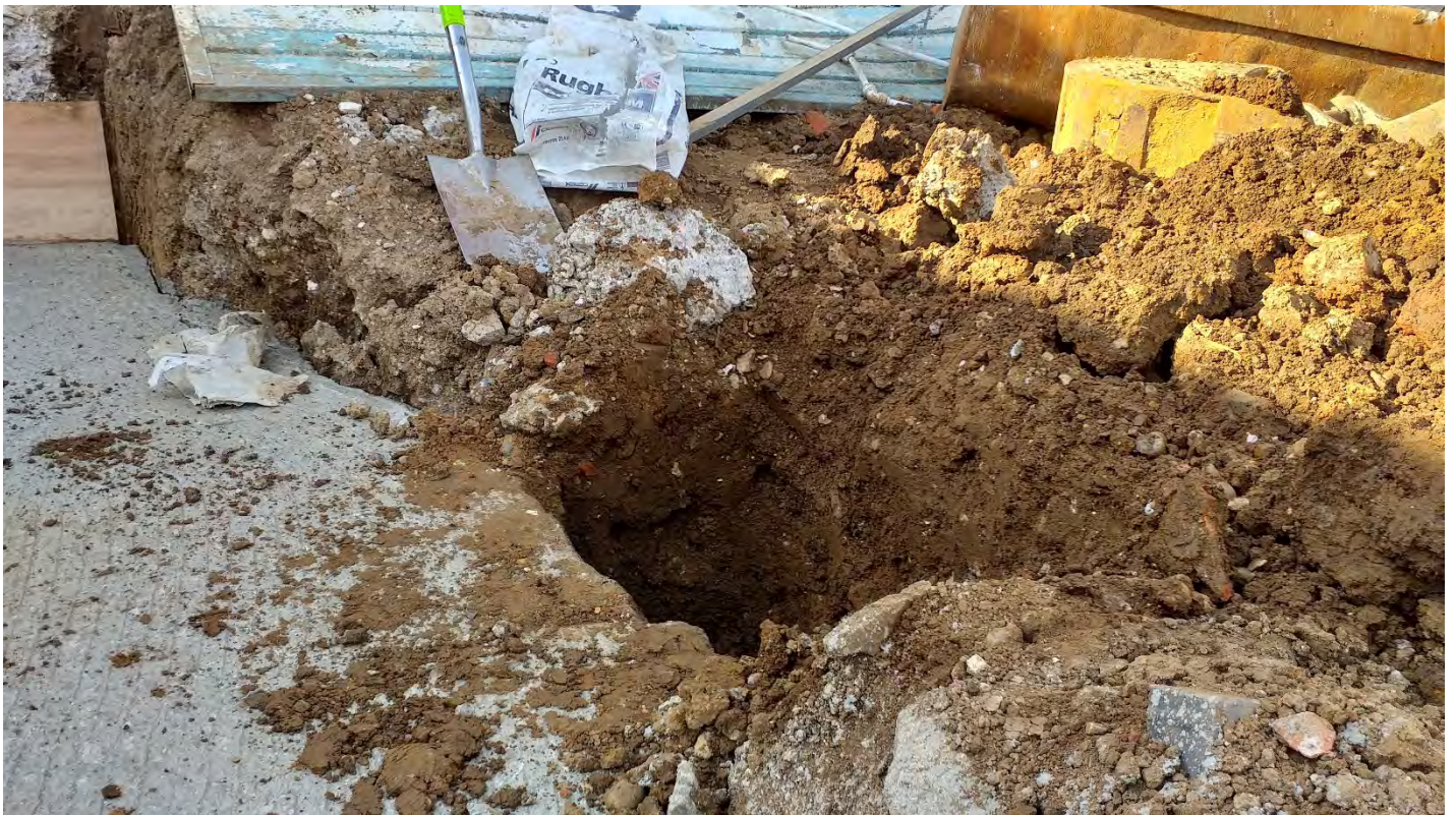
Above, re-excavation of the BH8 location (HD1)
