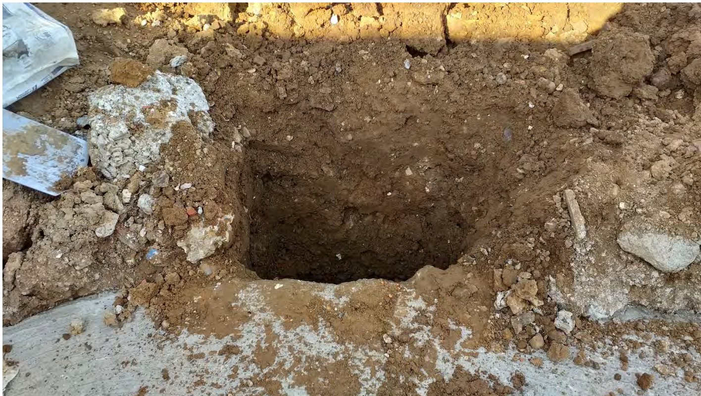
Above, re-excavation of the BH8 location (HD1)
