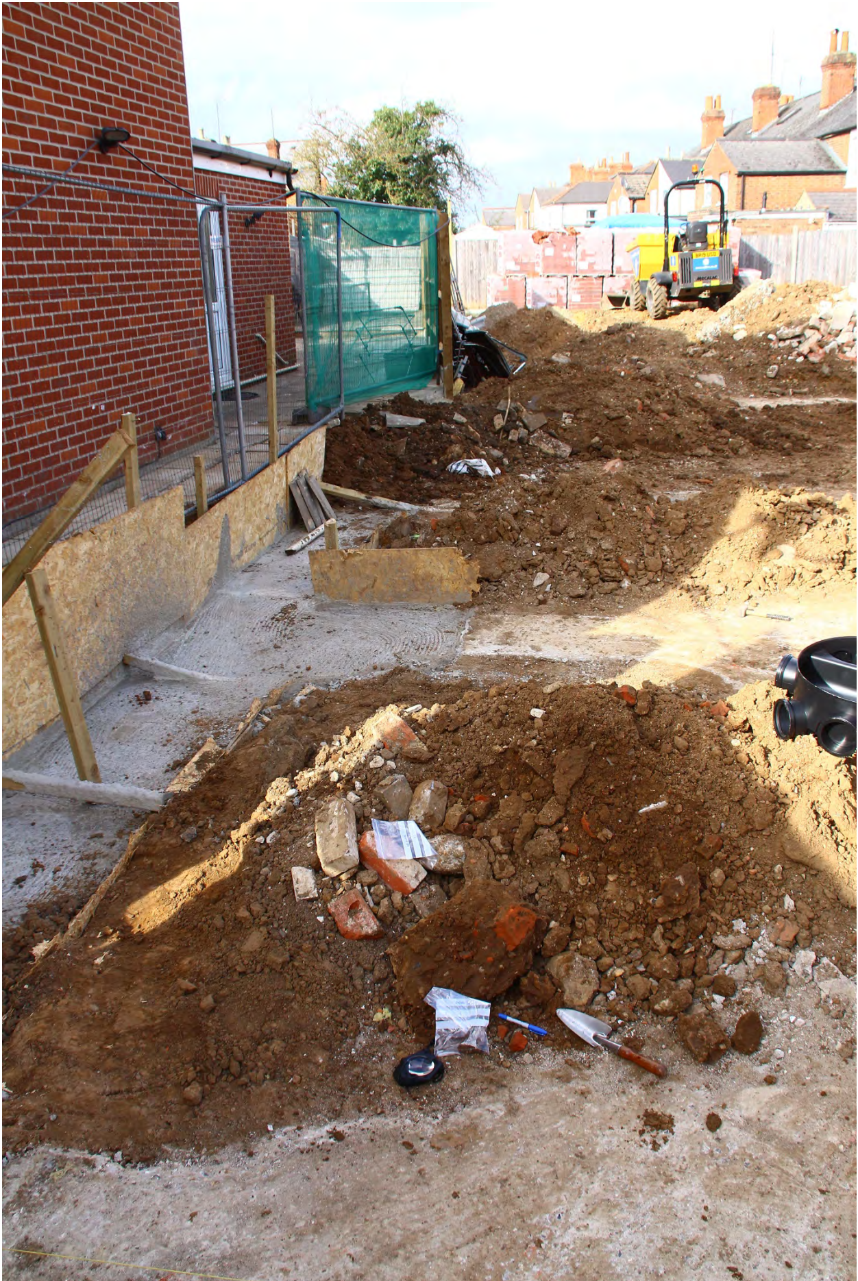
Above, a view looking north along the main section of the site
