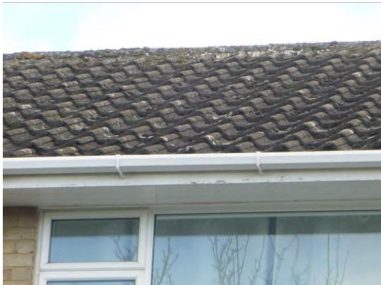
5. Ridge tiles in place and mortared.
