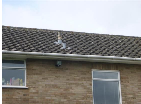
4. Interlocking roof tiles in place and tight on the roof.
