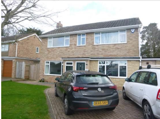
1. Front of the house viewed from the west.
