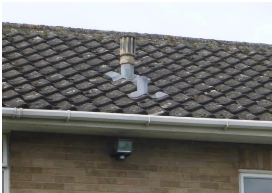
9. Lead flashing tight around the base of the flue pipe.
