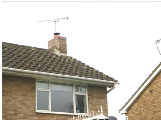
8. Lead flashing and new mortar tight around the chimney.
