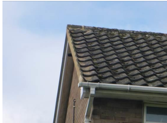
6. Newly mortared ridge tiles and verge tiles at the southern end of the roof.
