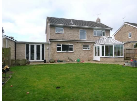
2. Rear of the house viewed from the east.
