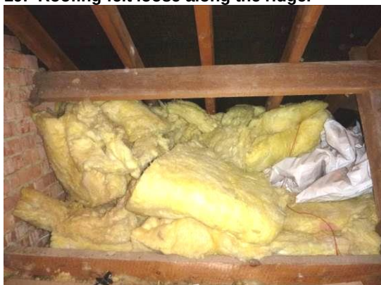
21. Roof lined with fibreglass and vermiculite.
