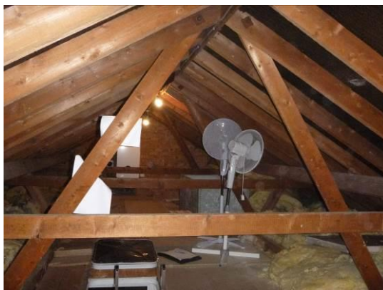
14. Internal view of the roof space.
