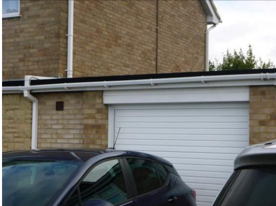
3. Flat roof extension to the front of the house.
