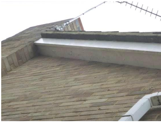
7. Verge fully mortared at the northern end of the house.
