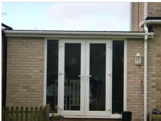
13. Flat roof covered tightly with bitumen roofing felt.
