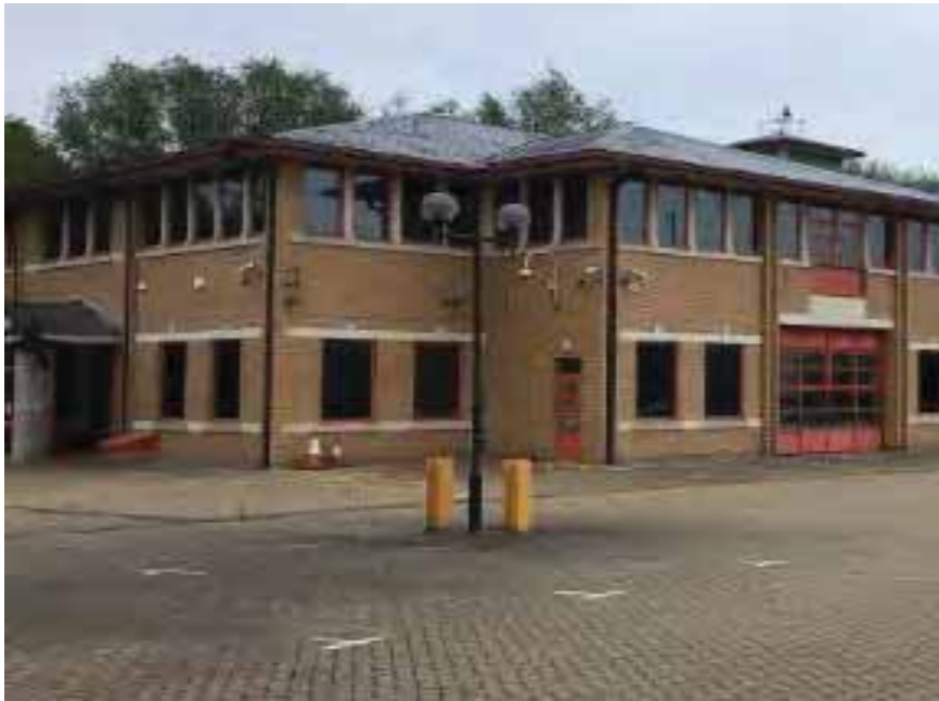
Photograph 1 View north-west towards southern end of the existing structure.
