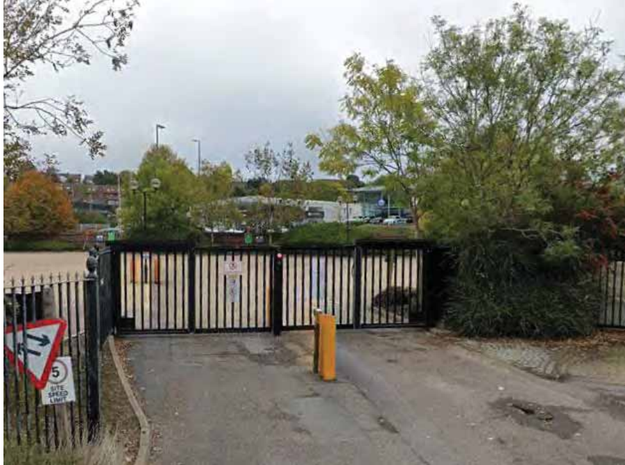
Photograph 5 Vehicular access to the south-western site boundary.
