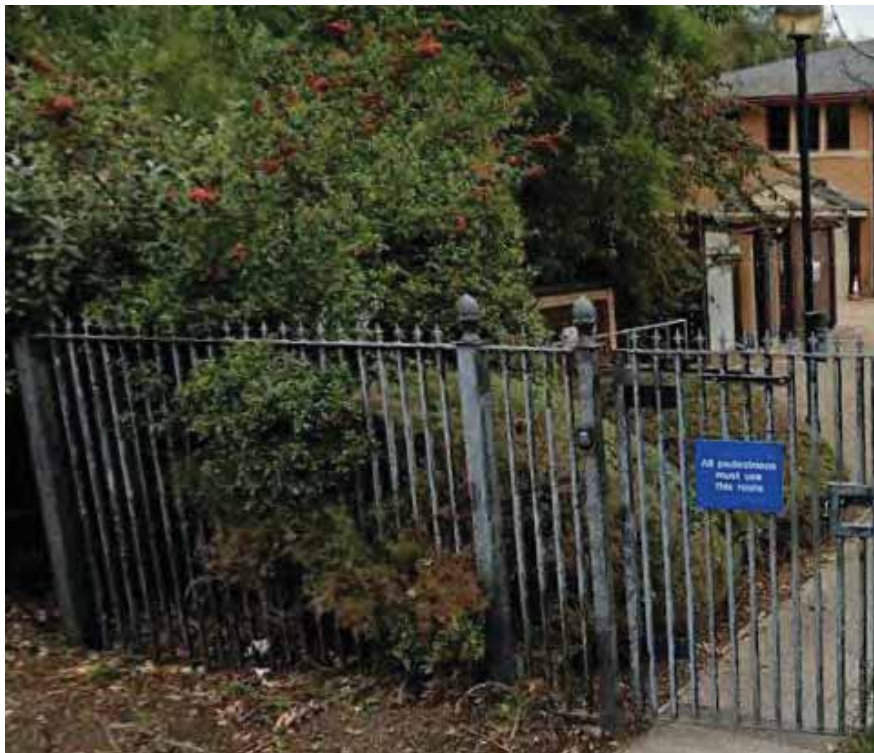
Photograph 4 Pedestrian gate into south-western site area with sub-station in the adjacent trees.
