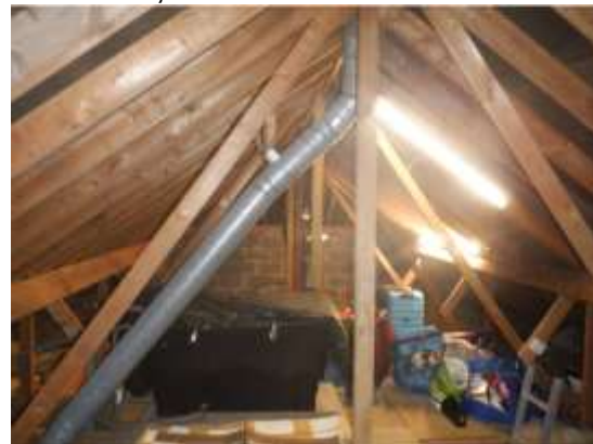
16. Cut and pitch roof construction.
