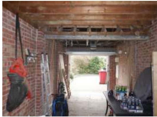
22. Garage with open roof space being used for storage.
