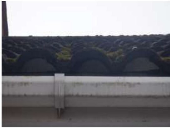
13. Open caps on interlocking tiles, viewed from the northeast.
