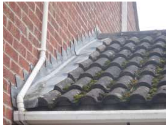
14. Lead flashing tight between garage and main house, viewed from the northeast.
