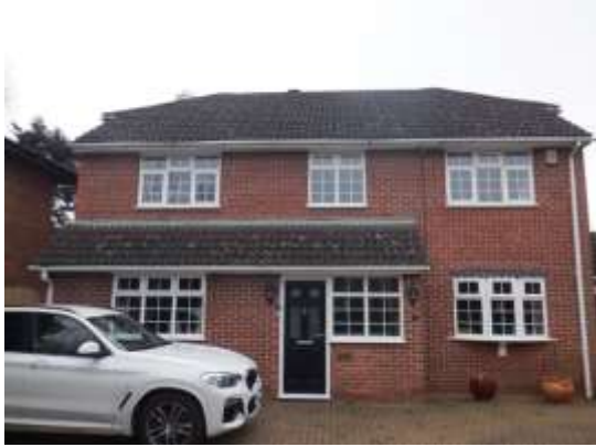
1. Front of the house viewed from the northeast.
