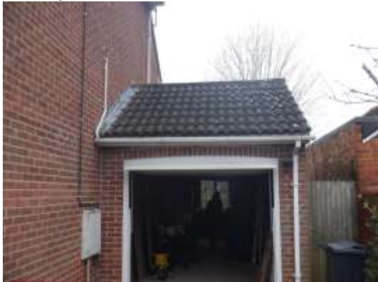
9. Front of the garage, viewed from the northeast.
