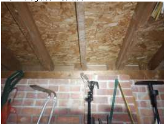
23. Wooden boarding on flat roofed section of the garage.
