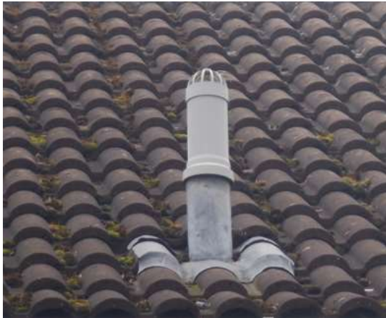
5. Lead flashing around the flue pipe tight to roof tiles, viewed from the southwest.
