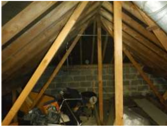
19. Stone block half-hipped gable end with soffit visible behind.
