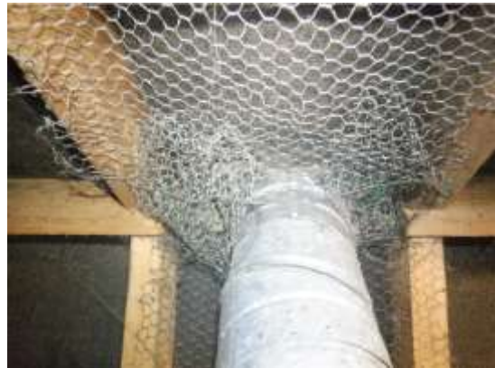
20. Large gap in bitumen felt with surrounding wire where pipe passes through
