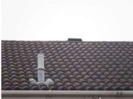
3. Tight interlocking tiles with a fully mortared ridge and vent brick, viewed from the southwest.
