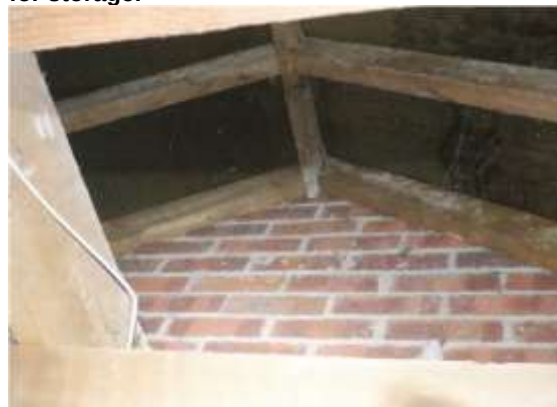
24. Timbers tight to the brick wall.
