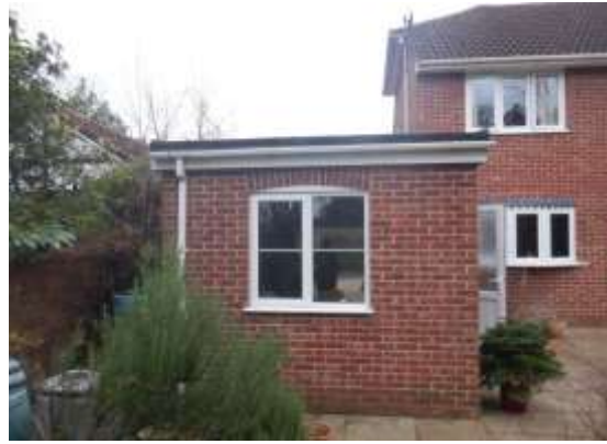
10. Rear of the garage, viewed from the southwest.
