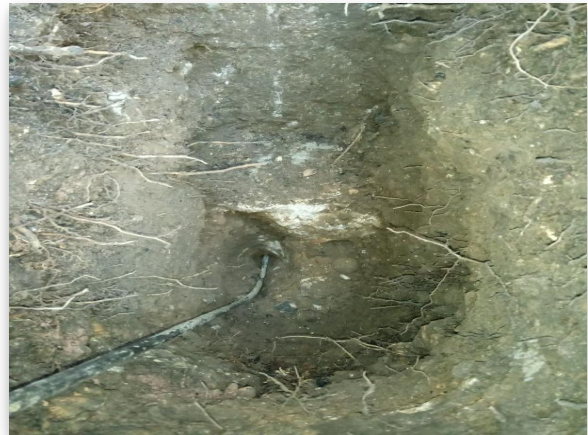
Fig 1.2: Trial Hole 1 Footing
