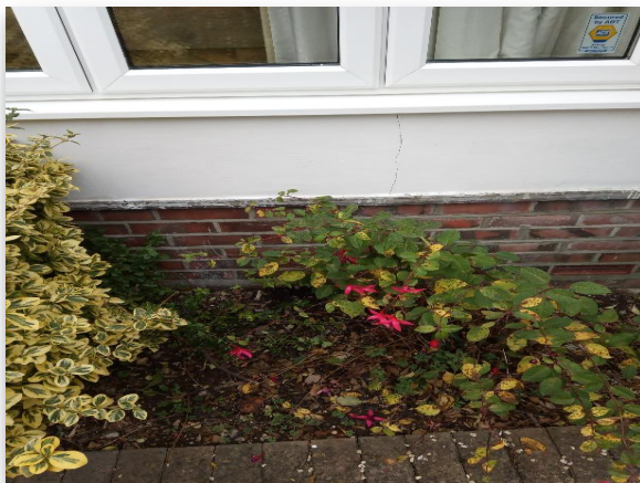
Fig 2.1: Trial Hole 2 Location
