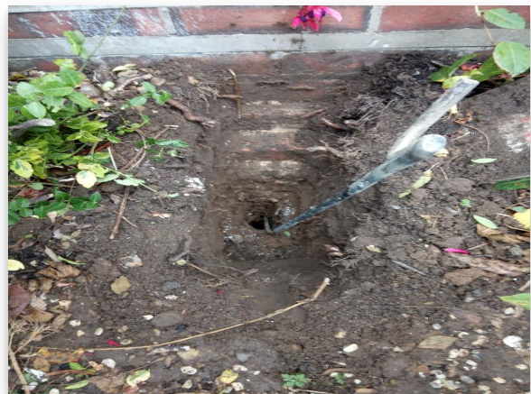
Fig 2.2: Trial Hole 2 Footing
