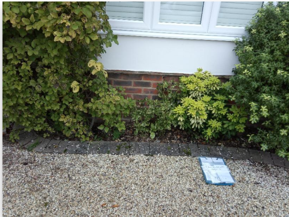
Fig 1.1: Trial Hole 1 Location
