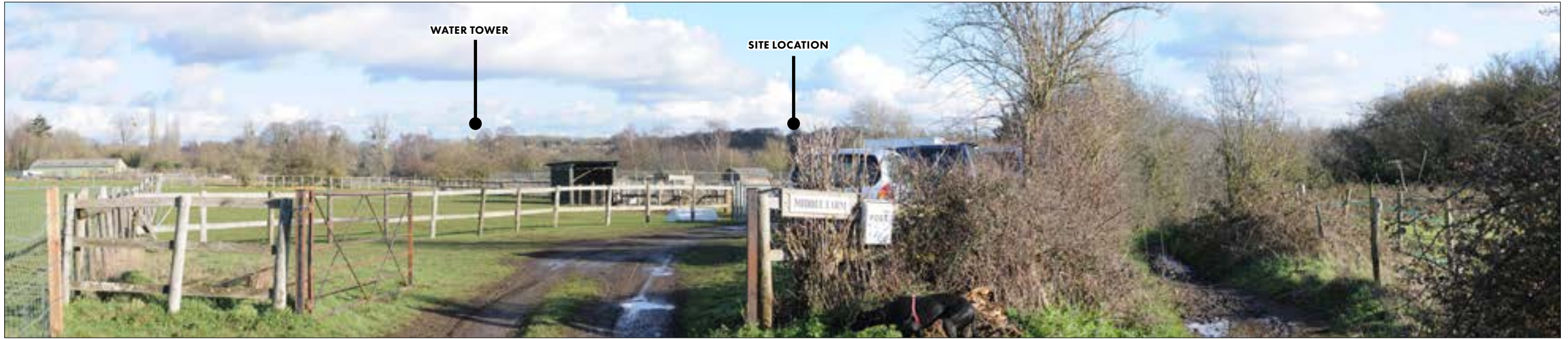
PHOTOGRAPH – VIEWPOINT 25 (WINTER 2019/2020) VALUE: LOW VIEW LOOKING EAST TOWARDS THE SITE FROM THE WESTERN BRIDLEWAY. THE WATER TOWER AND DWELLINGS SET AMONGST TREES ARE APPARENT. HOWEVER, THE VIEWS OF THE SITE ARE TRUNCATED BY THE INTERVENING VEGETATION.
