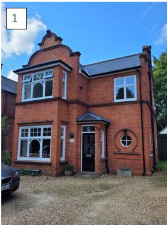
Figure 1: Photos of the site
